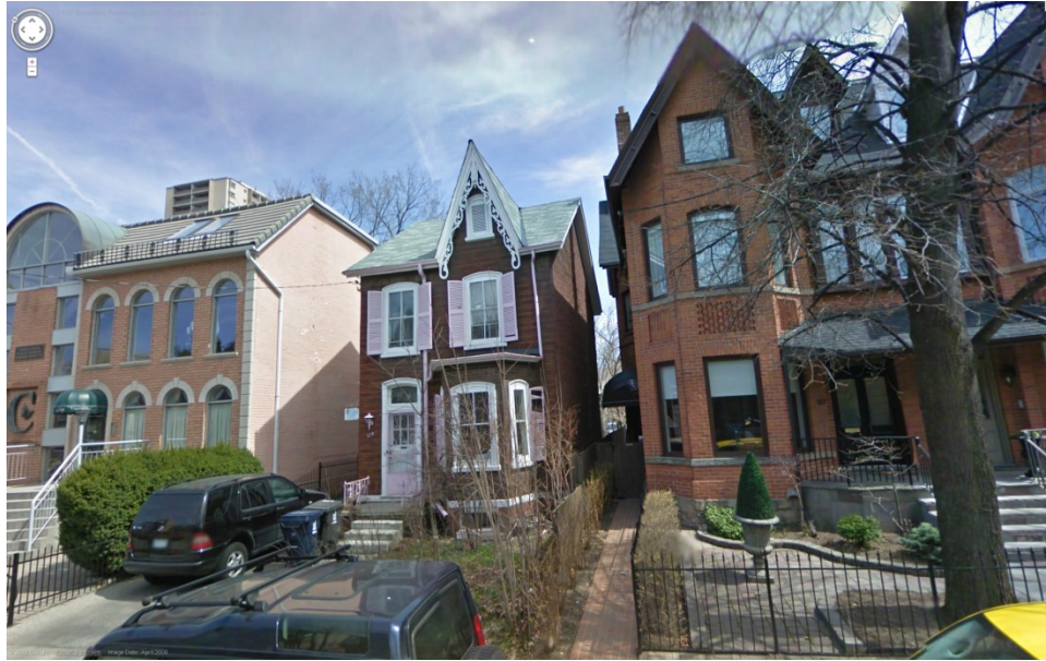
Context view of Hazelton Avenue prior to demolition of 131
