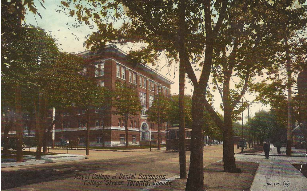
14. Archival Postcard, College and Huron Streets, 1913 : view looking east along College Street at Huron Street and showing the John Davison Buildings near the southeast corner of the intersection (right) (Toronto Historical Board)
