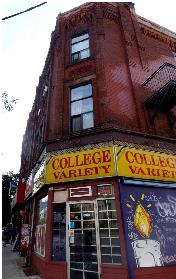
19. Current Photographs : showing the east elevation (above) and the beveled corner overlooking the intersection of College and Huron Streets (below) with the decorative terra cotta panel and corbelled brickwork (Heritage Preservation Services, September 2013)
