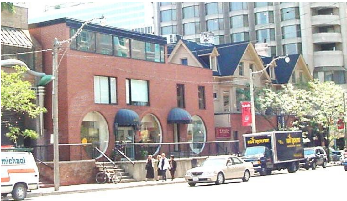
13. York Square, Three North Buildings on Avenue Road : the original buildings were completely refaced and a new third story added to two at the northern edge of the site. ( Heritage Preservation Services, October 2013 )
