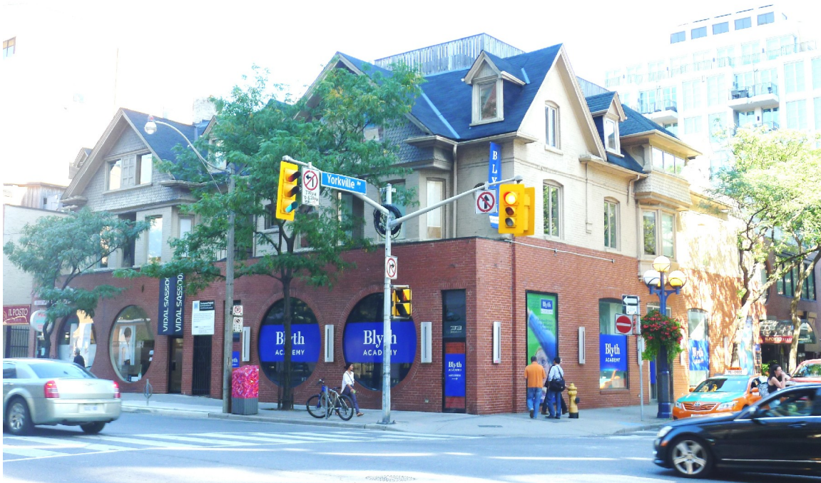
Principal (northwest) façades of York Square (Heritage Preservation Services, September 2013)
