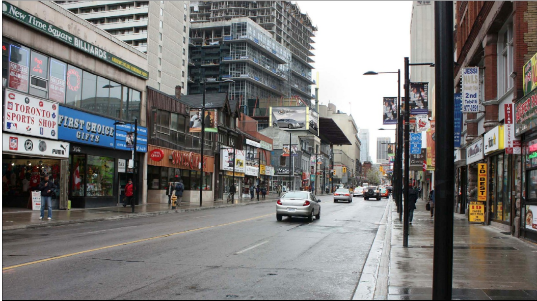
View Looking North on Yonge Street to Intersection of Gerrard and Yonge
