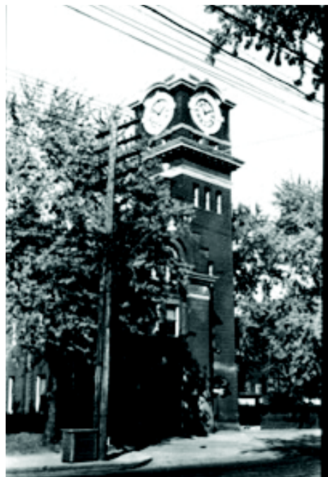
14. Kew Beach Fire Hall, 1952: note the presence of street trees in forecourt (Source: Toronto Reference Library Digital Archives).
