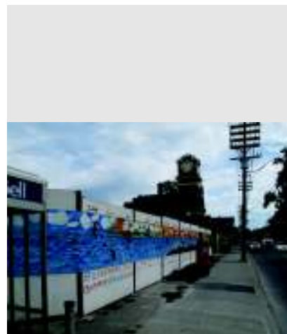
21. View of tower from north east corner of Queen St. E. and Woodbine Ave. (Source: ERA Architects Inc.).
