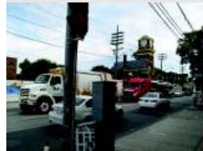
23. View of tower from south east corner of Queen St. E. and Woodbine Ave. (Source: ERA Architects Inc.).
