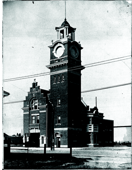
13. Kew Beach Fire Hall - Construction, 1905 (Source: City of Toronto Archives, Fonds 200, Series 372, Subseries 41, Item 803).
