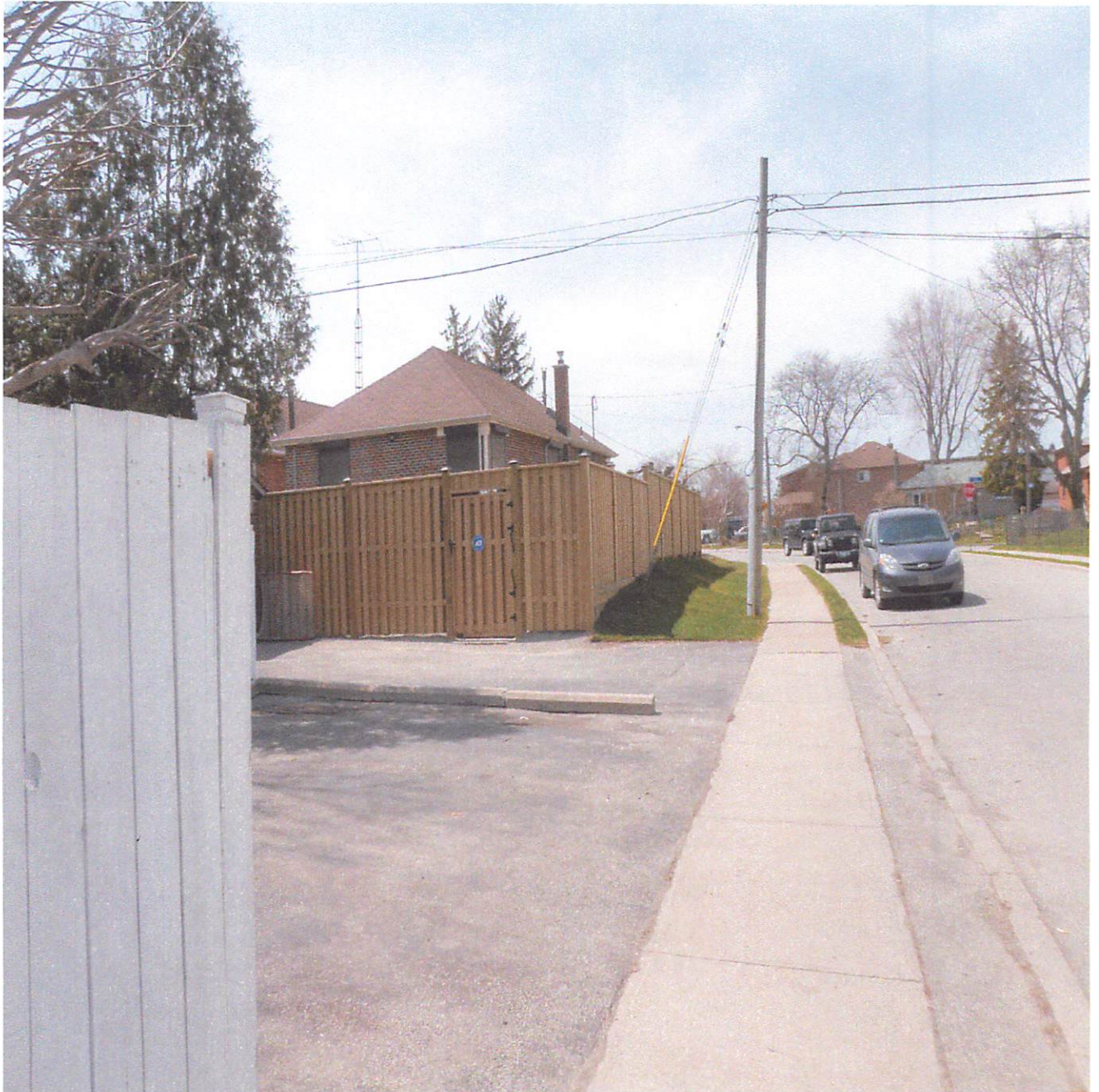
Photo 6 –looking west rear enclosure.
