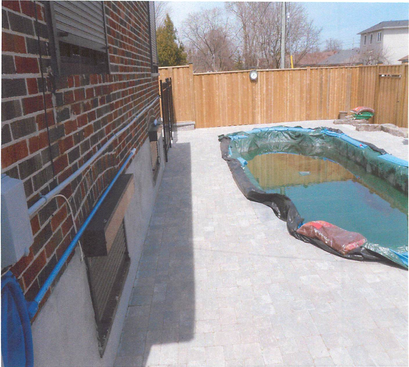
Photo 2- Rear yard no 4 th fence.
