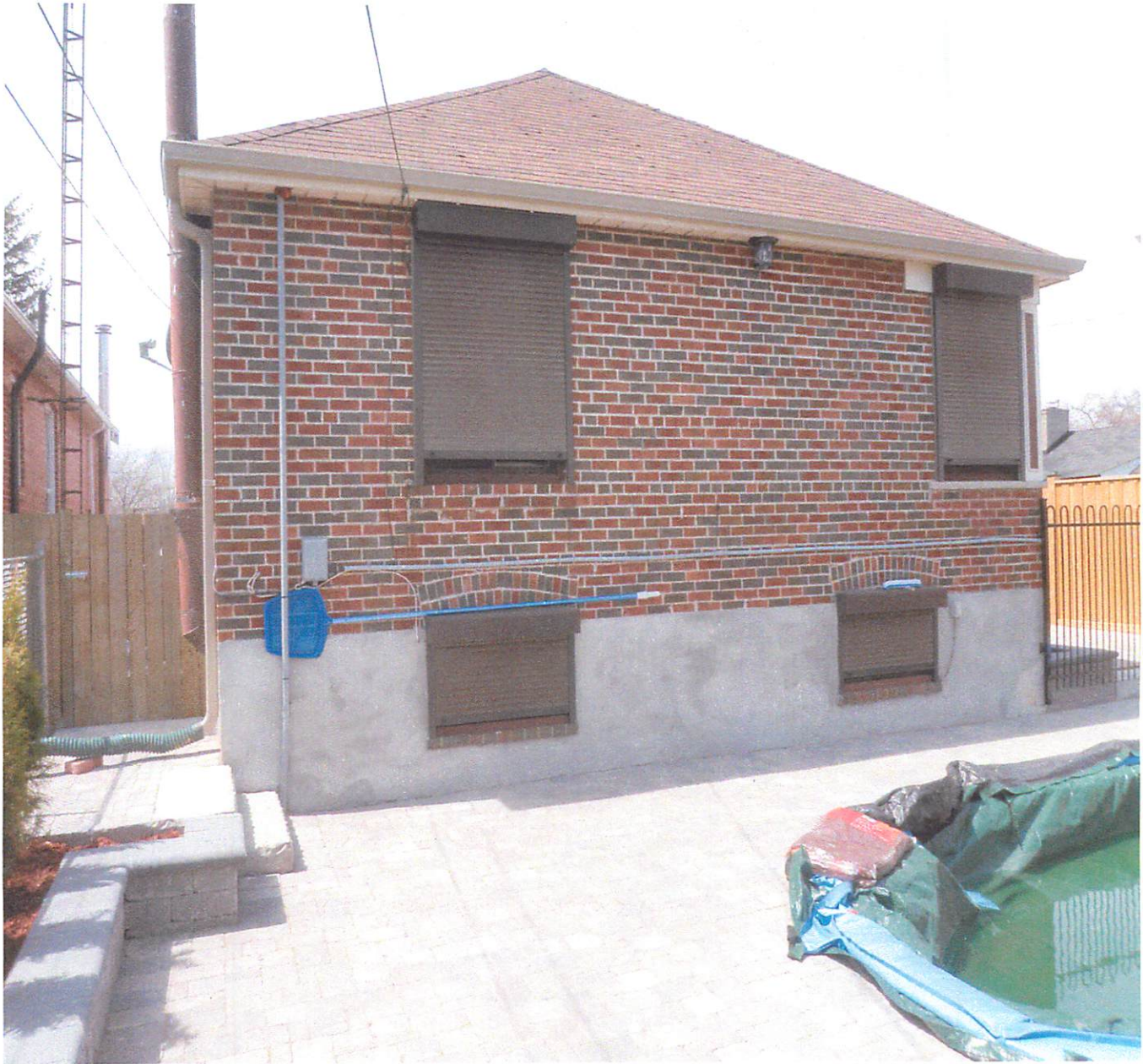
Photo 3- Rear Yard dwelling wall
