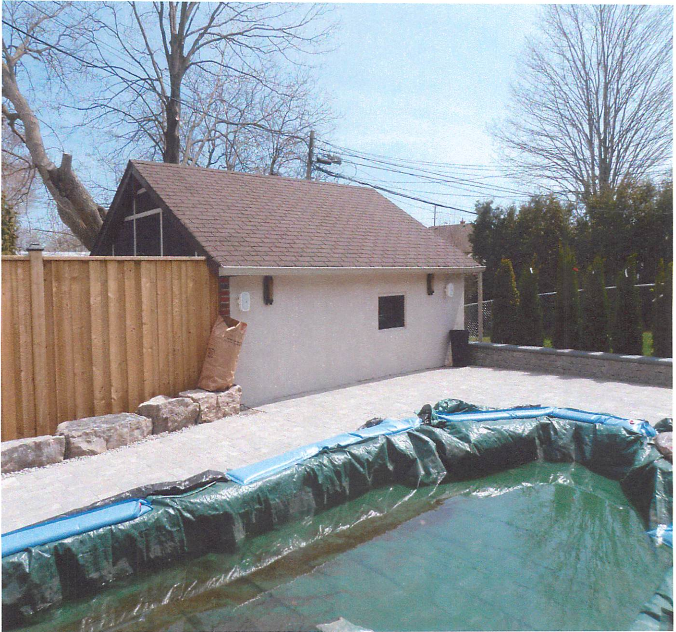
Photo 5- Rear garage wall opening window
