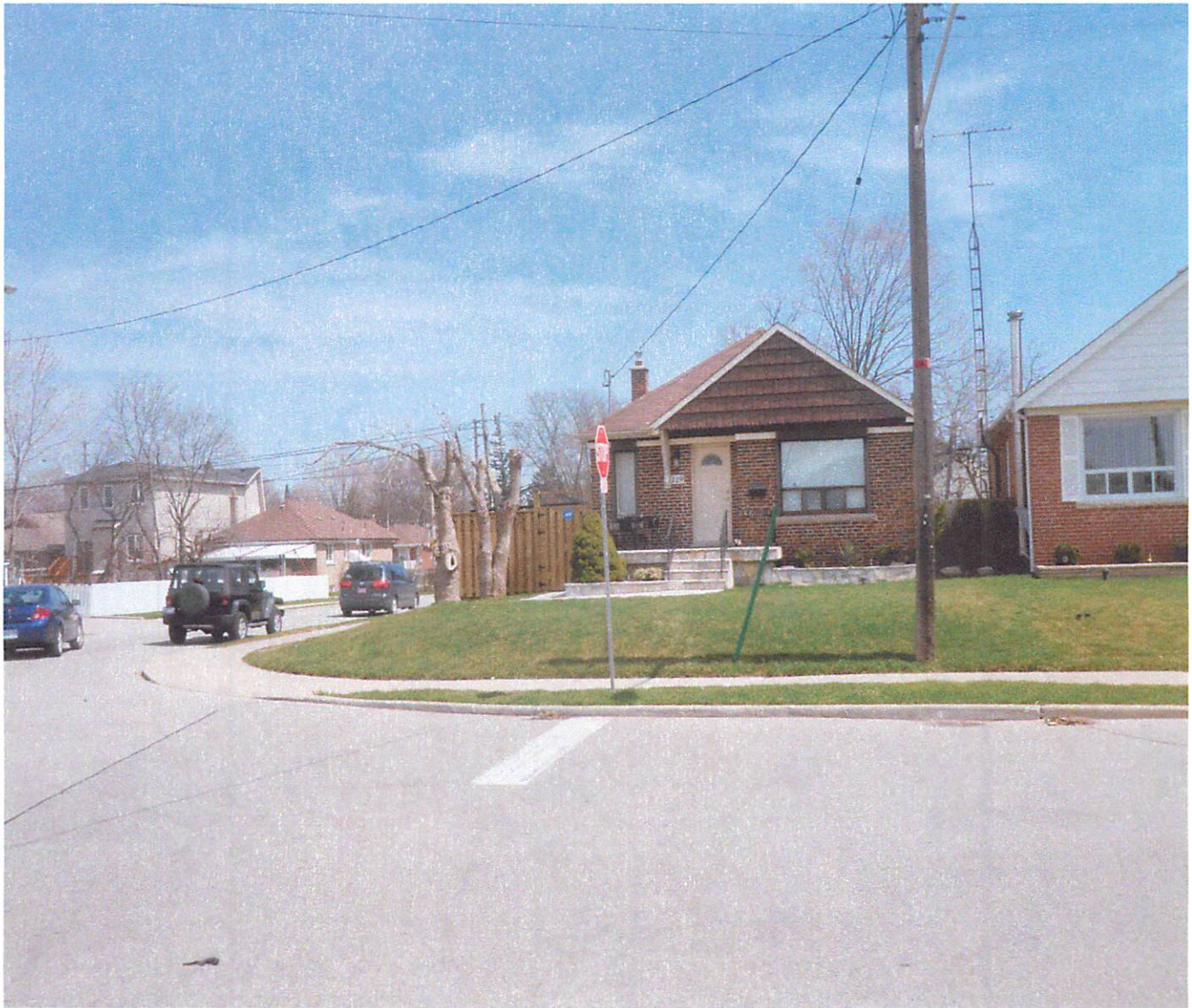
Photo 1- Front of property
