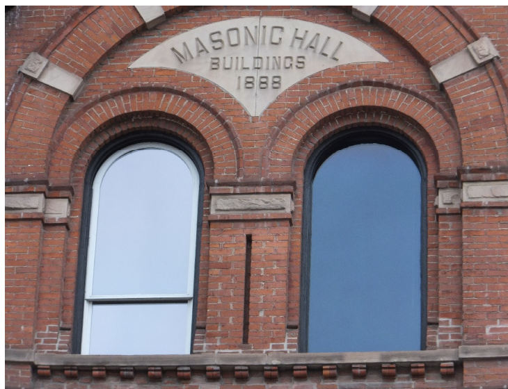
above: nameplate on west facade (Heritage Preservation Services, 2012)
