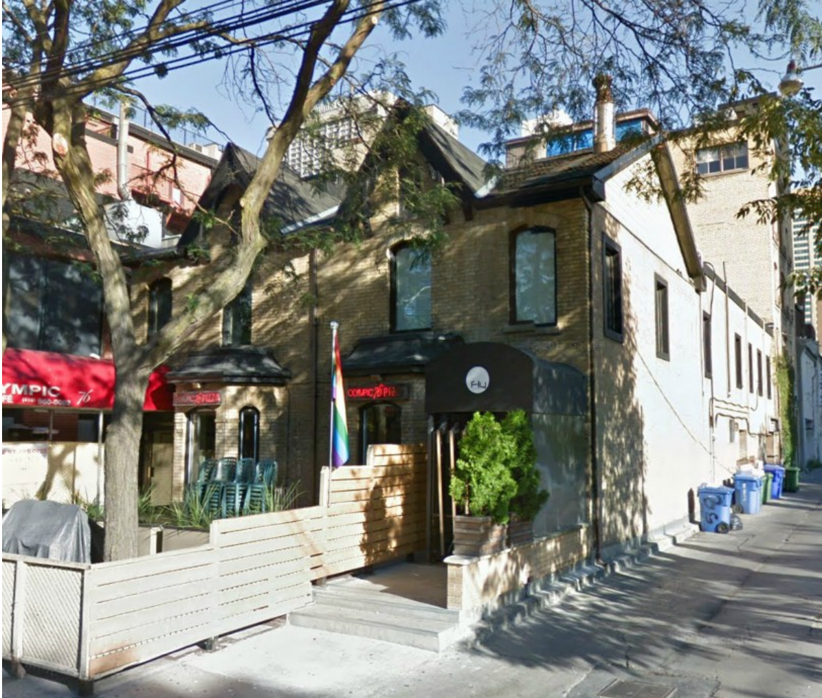
View from the South
