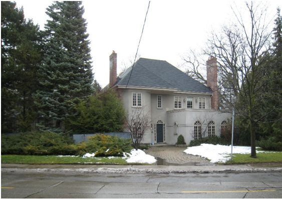
View of property from Glen Road
