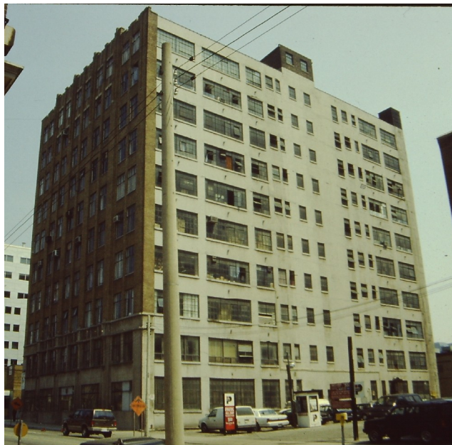
19. Archival Photograph, Commodore Building, 1991 : showing the west (left) and south (right) walls (Toronto Historical Board)
