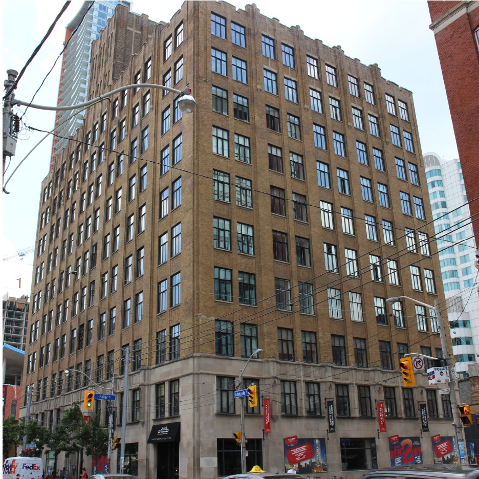
COMMODORE BUILDING 317 ADELAIDE STREET WEST, TORONTO
