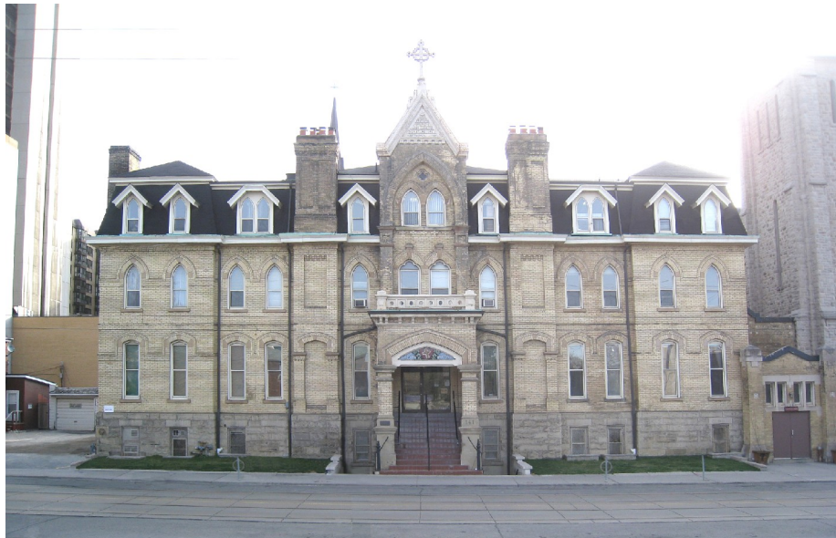
West Elevation, Redemptorists Monastery, 2013 (Stevens Burgess Architects)
