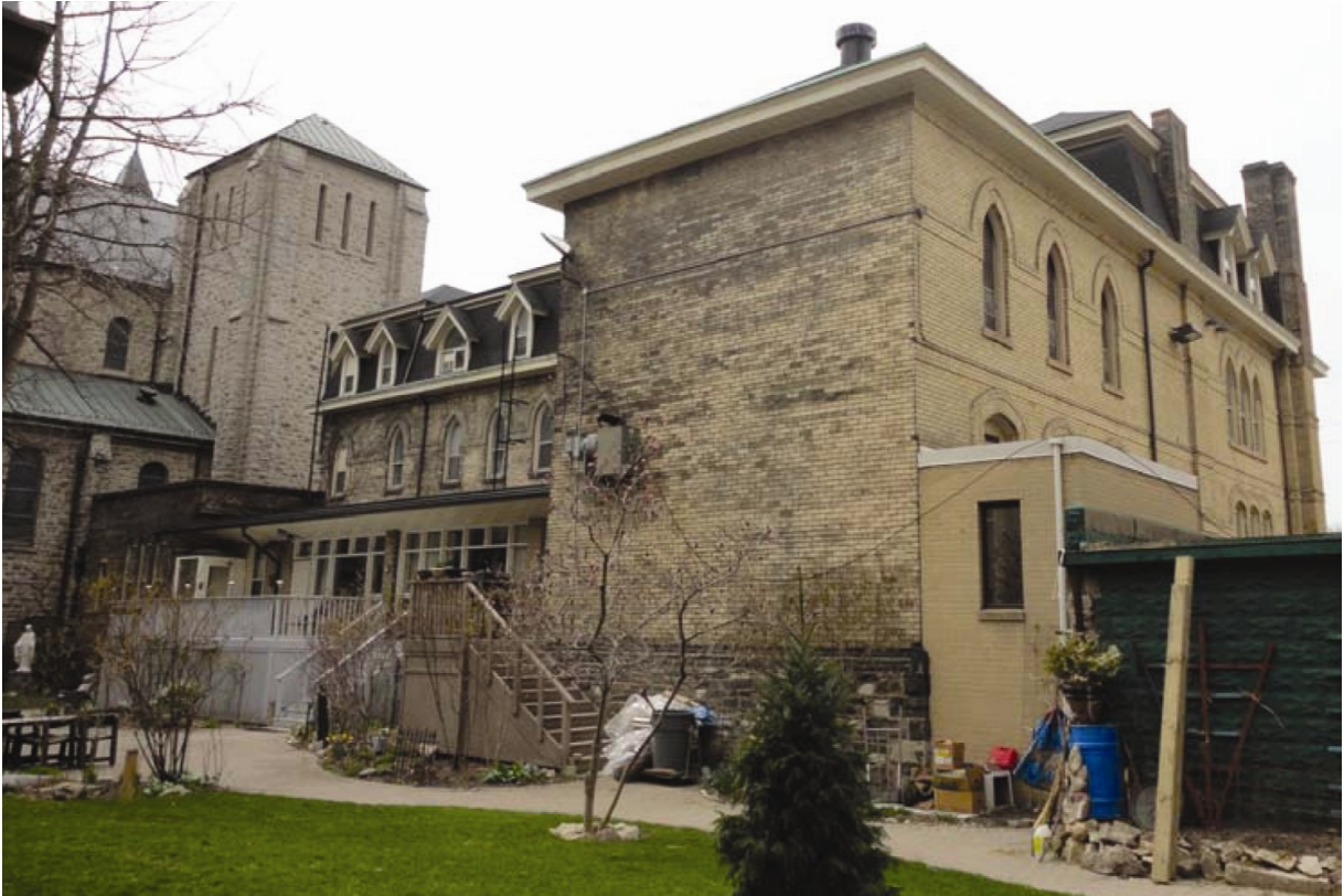
17. East Garden Side, St. Michael's Cathedral, 1989 ; showing the chapel wing with the later additions of the fire stairs on the right, the sun room and the extension to allow the link with St Patrick's Church (Stevens Burgess Architects)
