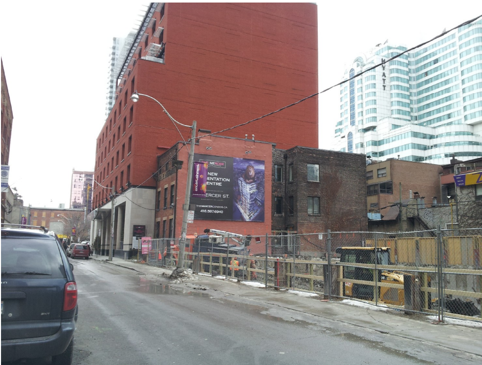
View of 24 Mercer Street showing south and east elevations
