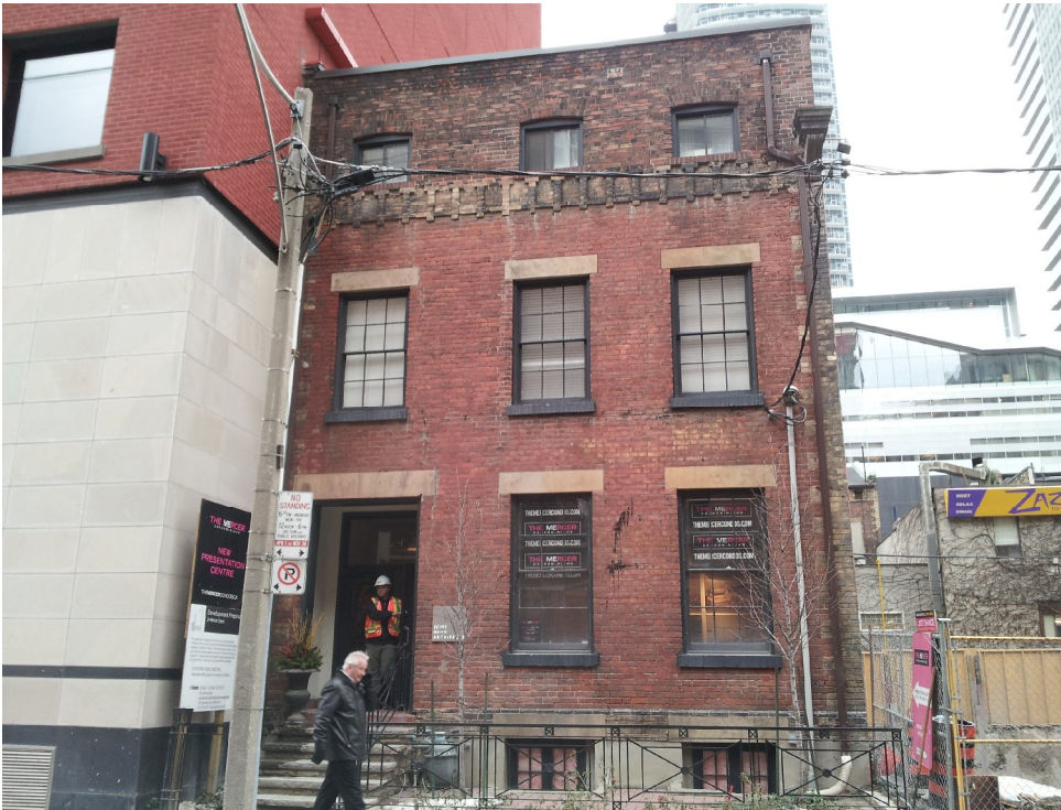
View of the primary elevation facing Mercer Street
