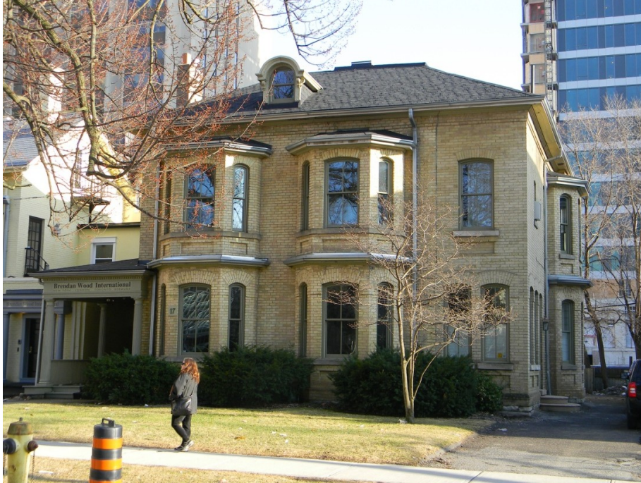
House pre-construction from the north-west
