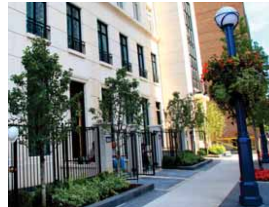
Interface between private yards and public boulevard
