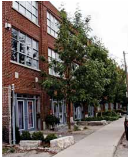
Enhance a narrow boulevard with planting in the setback area where possible
