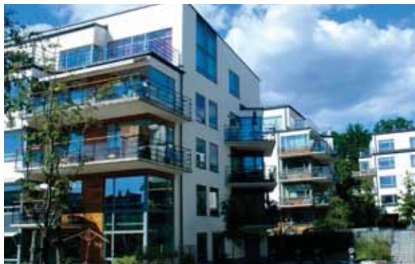
Apartments in Hammarby Sjostad, Stockholm
