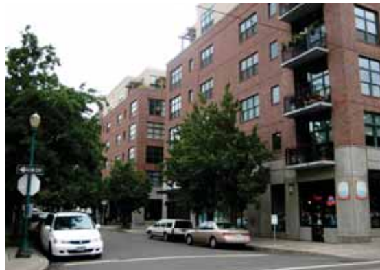
Apartments in Portland, Oregon
