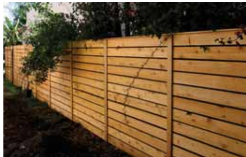
Backyards may have fences made of high-quality materials
