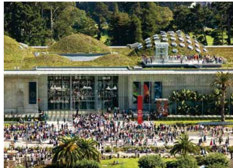
Green roof, California Academy of Fine Arts, San Francisco, California
