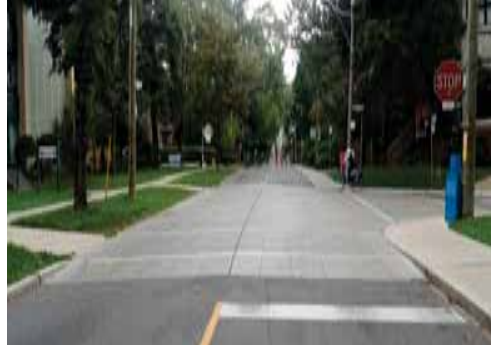
Key intersections may incorporate elements such as a traffic table, Heath Street, Toronto
