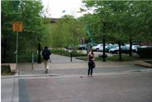
Depressed curbs, paving and signage identifies a pedestrian crossing, St. George Street, Toronto
