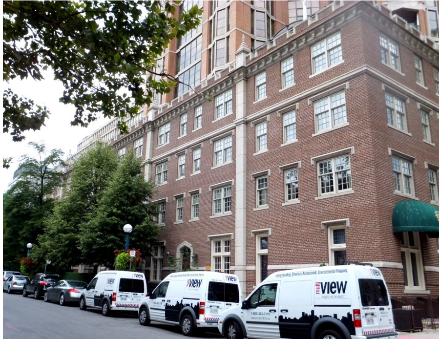
24. Current Photograph, Windsor Arms Hotel, 2013 : looking west from St. Thomas Street and showing the south elevation on Sultan Street
