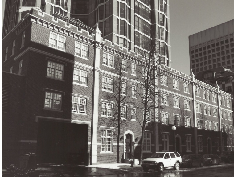
20. Photograph, Windsor Arms Hotel, 2000: showing the south elevation on Sultan Street with the entrance to the parking garage (left) (Heritage Preservation Services)
