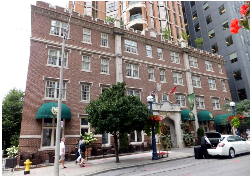
22. Current Photograph, Windsor Arms Hotel, 2013 : showing the principal (east) facade (Heritage Preservation Services)
