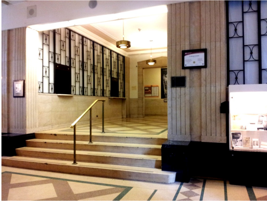
26. Photograph, Lobby, E-wing, St. Michael's Hospital, 2013: looking north and showing the stairs and corridor at the north end of the lobby, which continues the decorative detailing and materials (Heritage Preservation Services)
