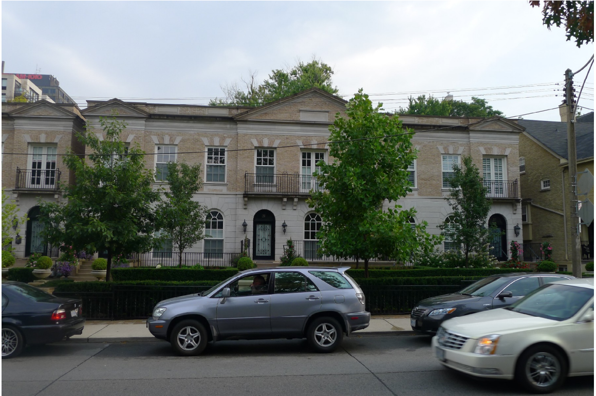
12. 27-33 Heath Street, late 20thc. (Heritage Preservation Services, August 2013)
