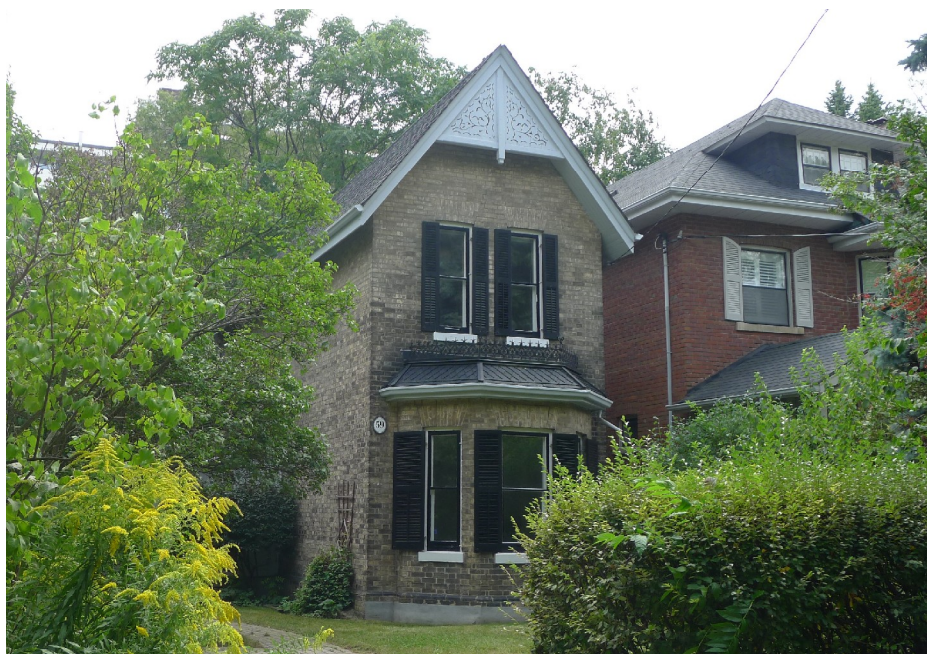
Principal (north) façade of 59 Heath Street West (Heritage Preservation Services, September 2013)
