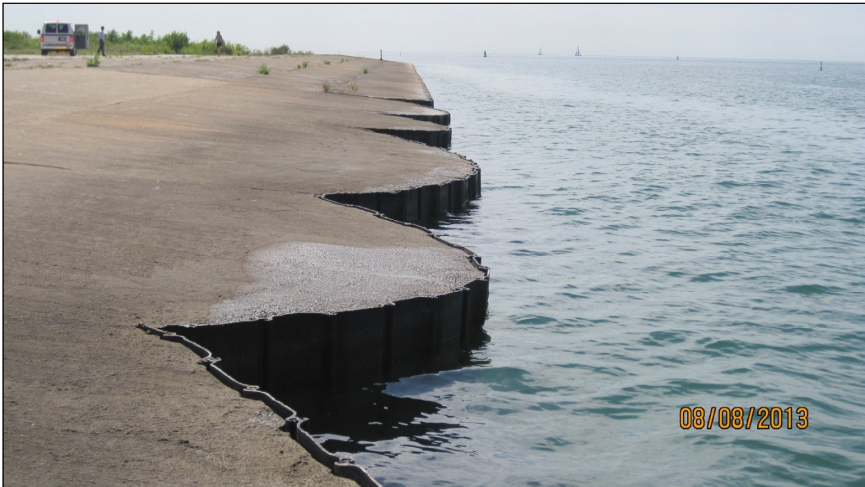
Figure 3-8 View South of the Northeastern Cellular Quay
