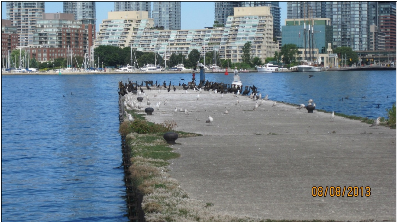
Figure 3-4 Moss and Lichen on the Northeastern Pier
