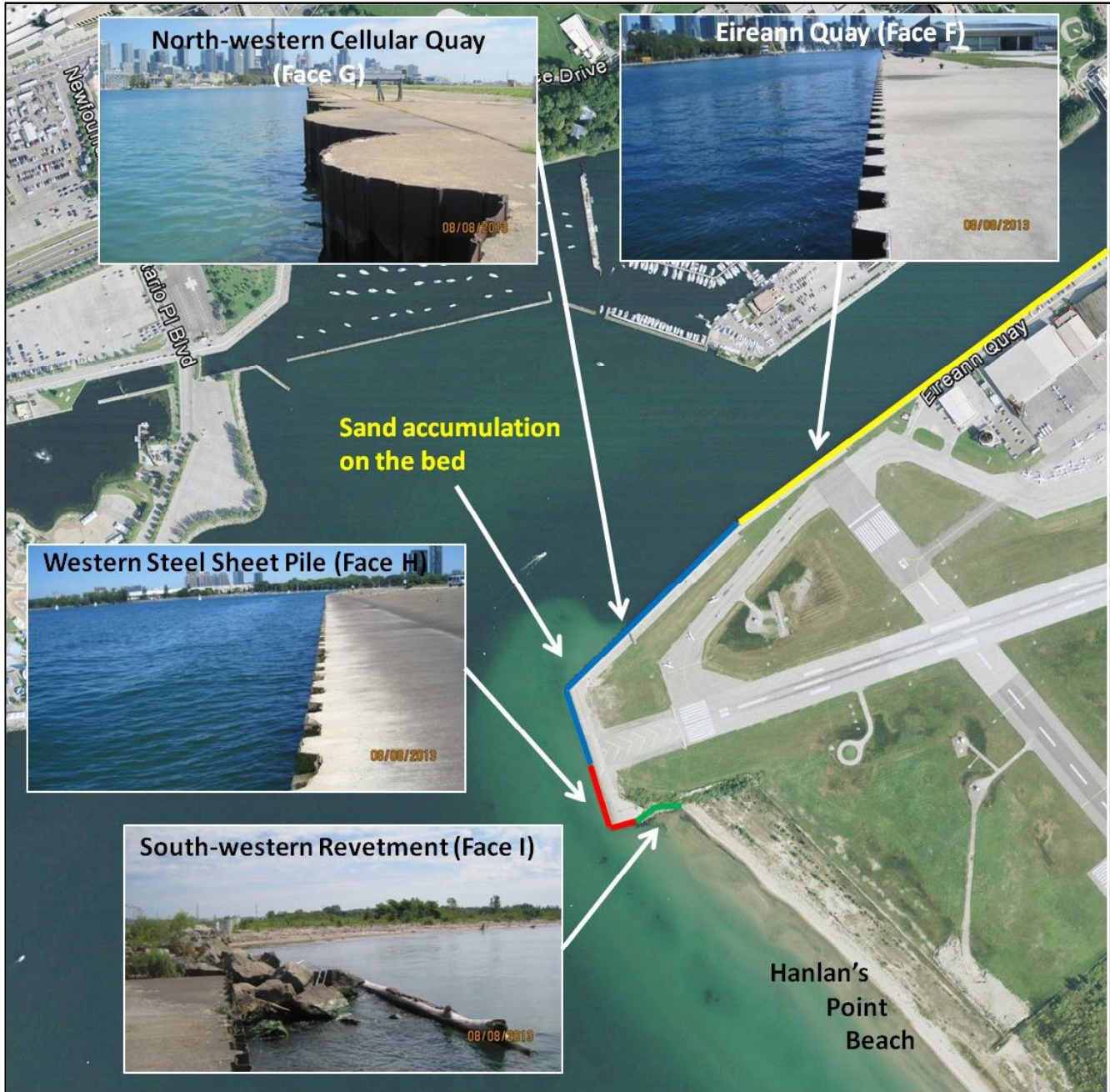
Figure 3-6 Existing Shoreline Conditions on the Western Runway
