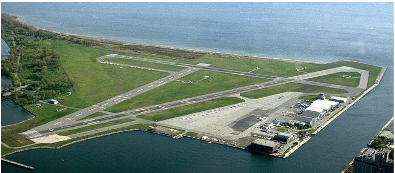
Aerial view of the Billy Bishop Toronto City Airport
