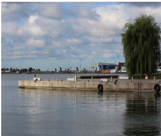
Wharf at HTO Park West
