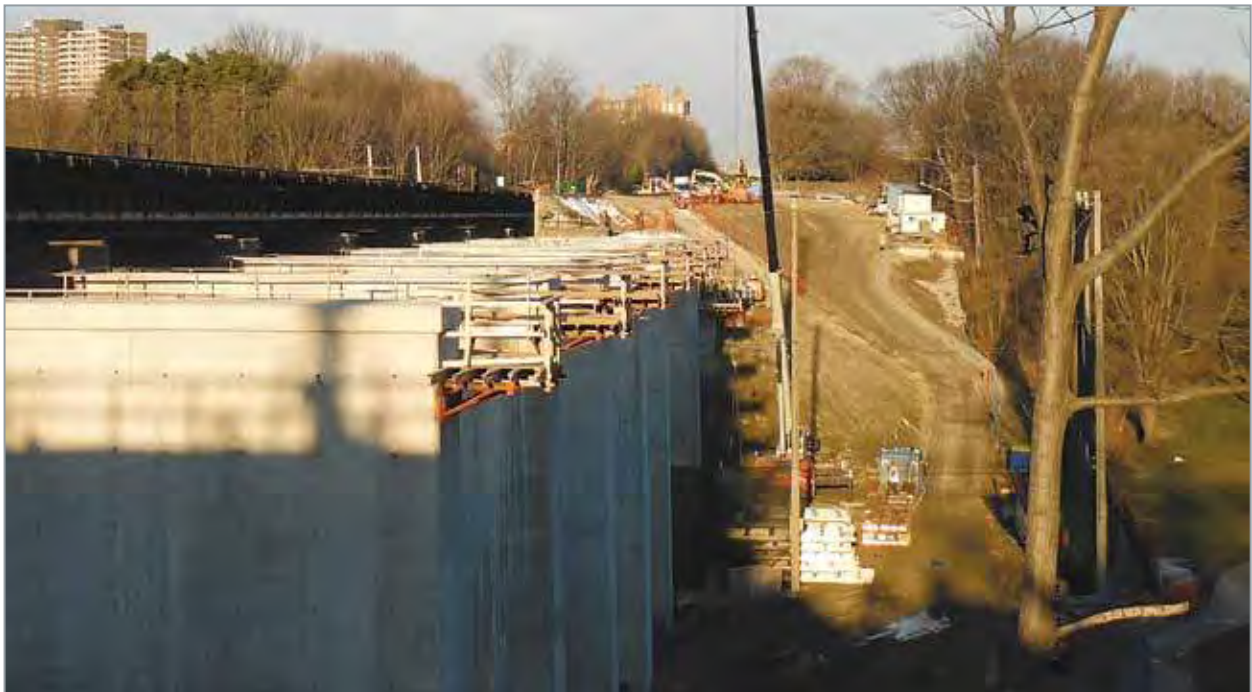
Viaduct widening at the Humber River, part of GO Transit's Georgetown South Project
