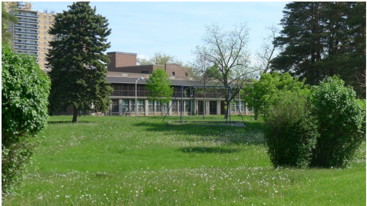
16. Photograph from the south west on the driveway looking north east to the south face of the hospital patient's wing: showing mature planting and lawns (Heritage Preservation Services, June 2014)
