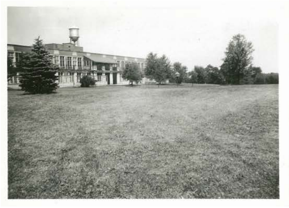
15. Photograph from the south west looking north east to the south face of the hospital patient's wing: showing the development of the lawns and planting (Hospital Archives, The Hospital for Sick Children, Toronto)
