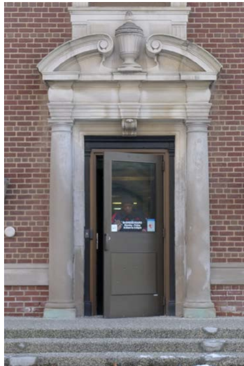
6. North Façade, Main Entry Door Case: with the classical elements of the Tuscan Doric columns, broken pediment flanking an urn and decorative entablature with bulging frieze above and volute bracket (Heritage Preservation Services, December 2013)
