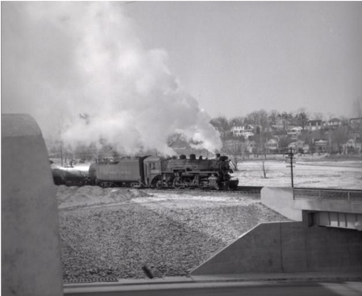
C.P.R. tracks, looking w. over Royal York Rd.
