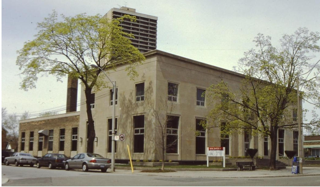
23. Photograph, Postal Station “K”, 1996 : showing the east façade and south elevation on Helendale Avenue (Toronto Historical Board)
