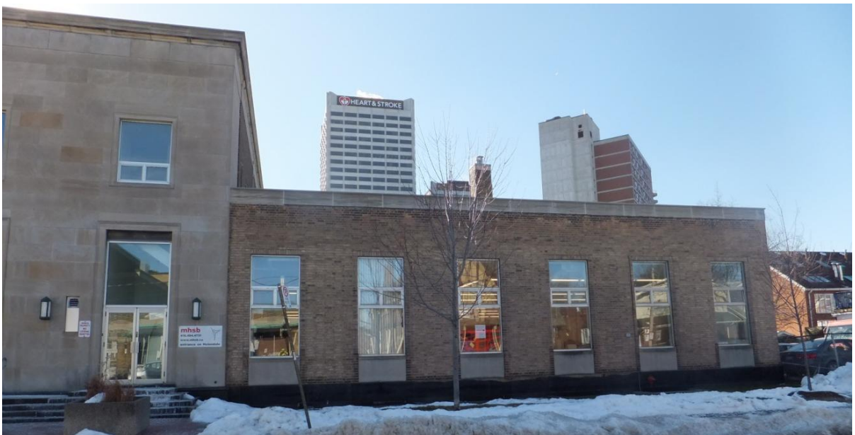
26. Photograph, 2384 Yonge Street, 2013 : showing part of the north elevation on Montgomery Avenue with the sorting station on the right (Heritage Preservation Services)
