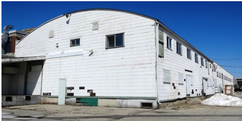
Building 38 (above) and Building 39 (below) (Heritage Preservation Services, March 2014)
