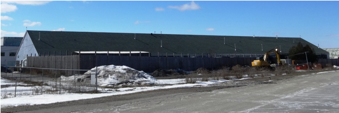
Building 42 (Heritage Preservation Services, March 2014)
