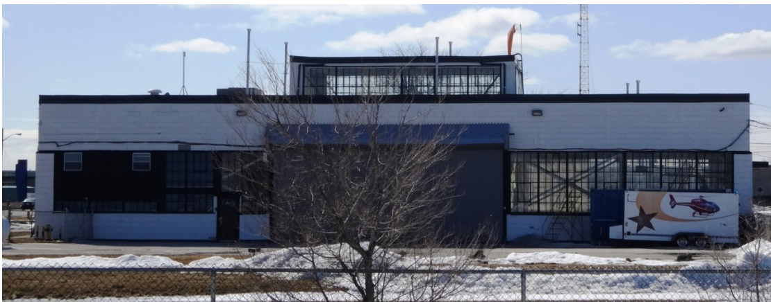
Building 43 (Heritage Preservation Services, March 2014)
