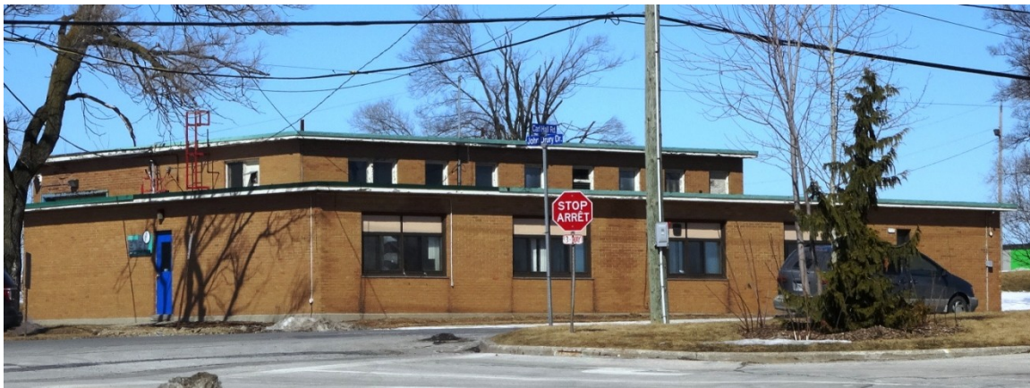
Building 103 (Heritage Preservation Services, March 2014)
