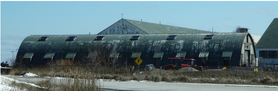
Building 41 (Heritage Preservation Services, March 2014)
