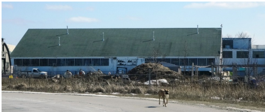
Building 40 (Heritage Preservation Services, March 2014)
