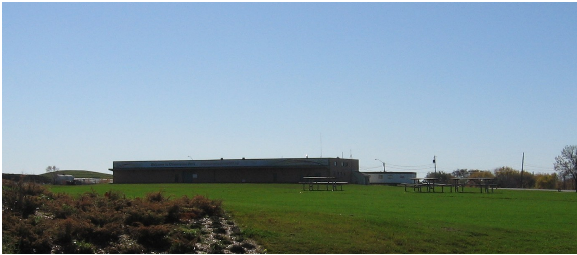
Building No. 106: Guard House and Storage Building (1953)
