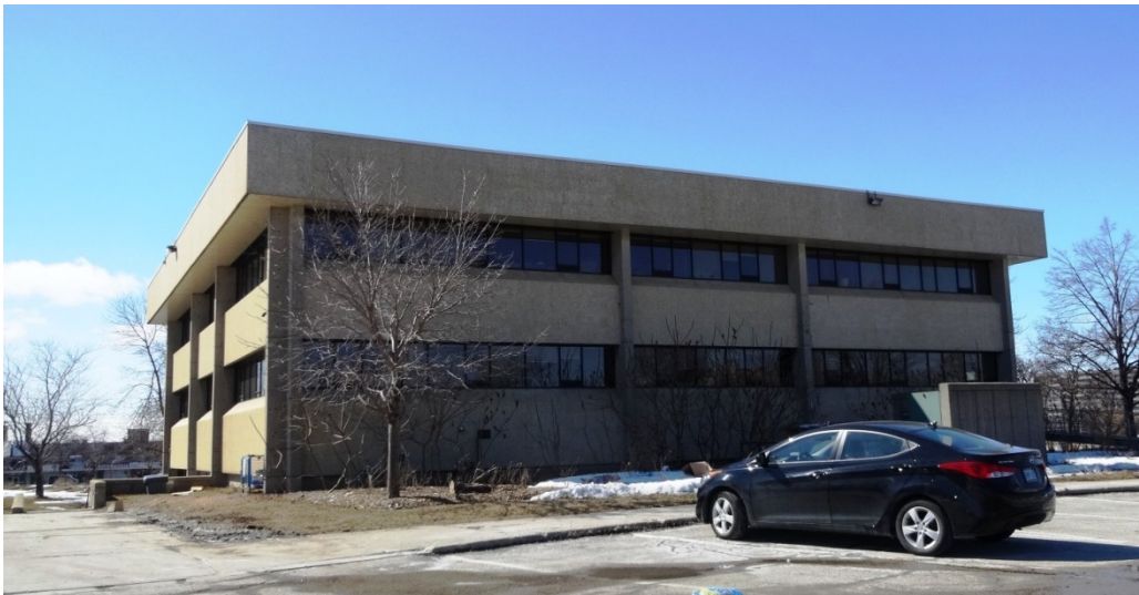
Building 100 (Heritage Preservation Services, March 2014)
