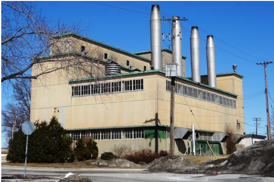
Building 105 (Heritage Preservation Services, March 2014)
