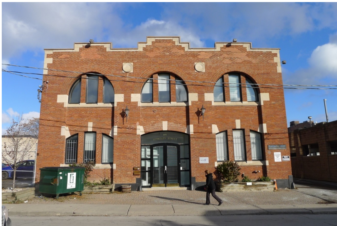
Principal (west) façade of the Christie, Brown & Co. Stables (Heritage Preservation Services, December 2013)
