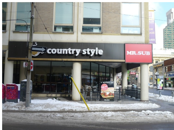
10. Corner of Yonge and St. Mary streets showing the set back of the glass façade to create an open volume at the base of the building. (Heritage Preservation Services 2014)
