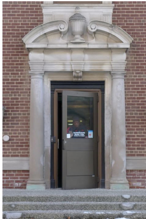
6. North Façade : Main Entry Door Case: with the classical elements of the Tuscan Doric columns, broken pediment flanking an urn and decorative entablature with bulging frieze above and volute bracket (Heritage Preservation Services, December 2013)
