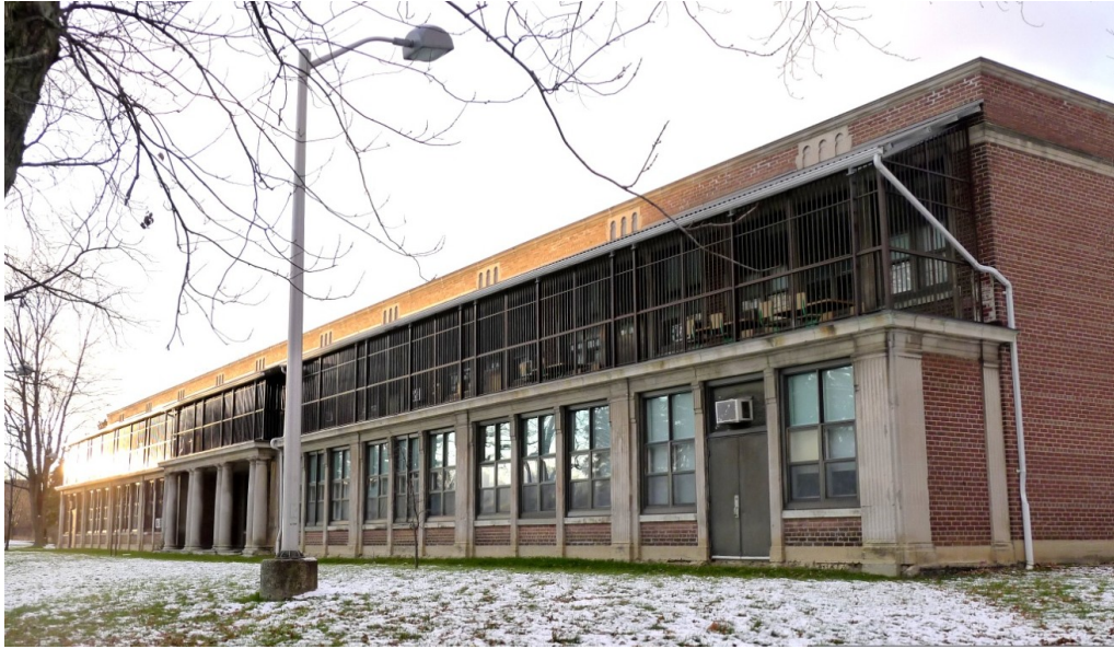
Above: South façade of the former Sick Children's Hospital (County Branch) Thistleton, now the Thistleton Regional Centre for Children and Adolescents (HPS 2013)
