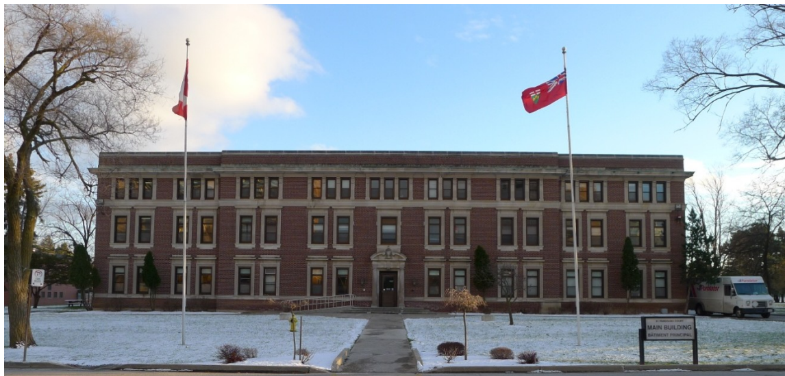
Principal (north) façade of the former Sick Children's Hospital (County Branch) Thistletown, now the Thistletown Regional Centre for Children and Adolescents (Heritage Preservation Services, December 2013)
