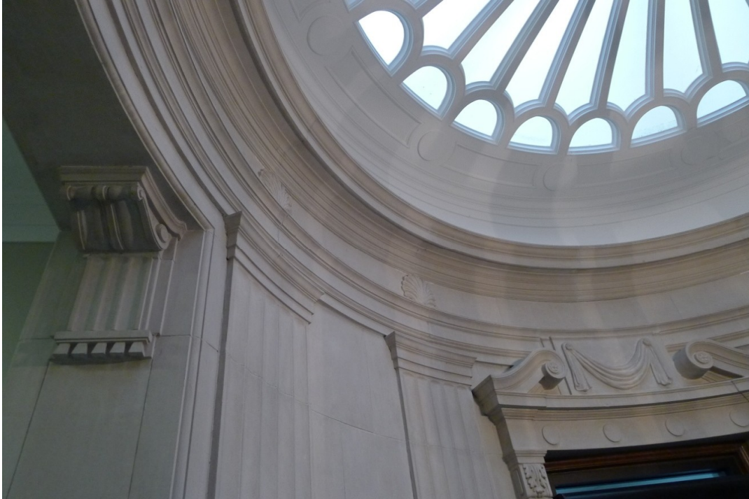
10. Rotunda Details : Caen stone details including fluted pilasters, door cases and brackets and the tracery details of the skylight (Heritage Preservation Services, December 2013)
