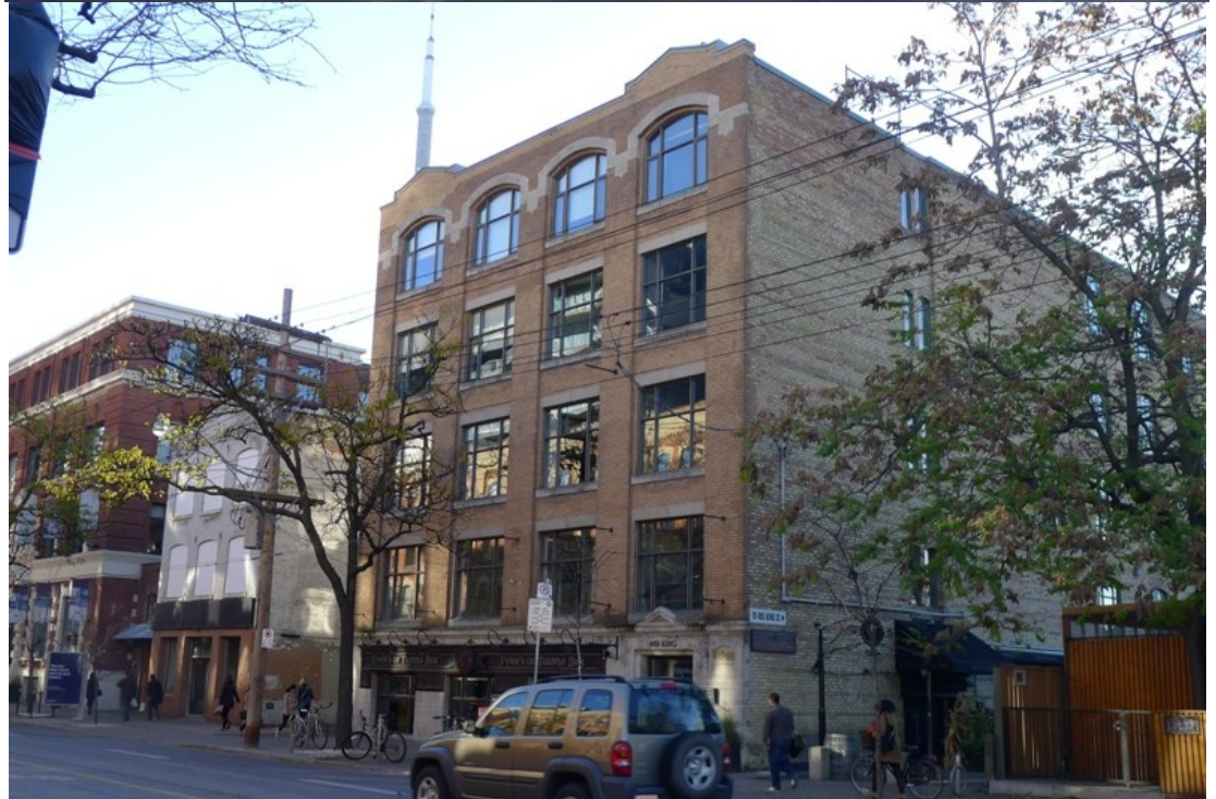
Hart Building, principal, north façade (above) and context (below) on King Street West (Heritage Preservation Services)
