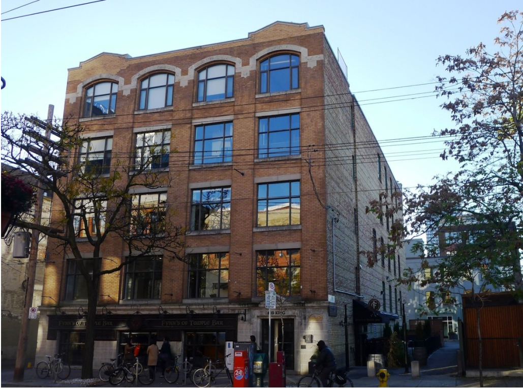
7. Hart Building, 489 King Street West : principal façade (Heritage Preservation Services, November 2013)
