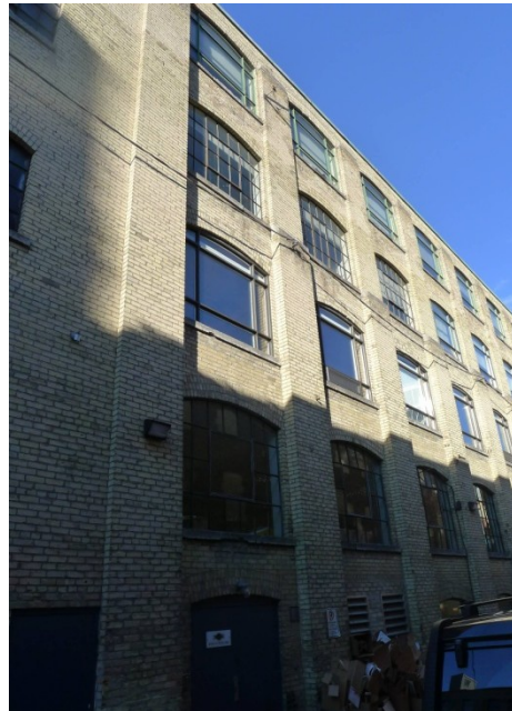
10. Hart Building, 489 King Street West : showing the east façade with the stone-capped stepped buttresses and varying window glazing (Heritage Preservation Services, November 2013)
