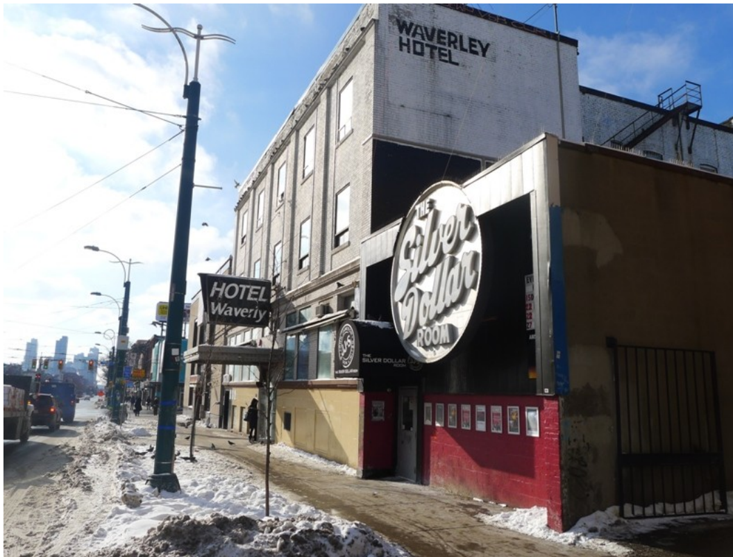
Principal (east) façades of 484 Spadina Avenue, the Waverley Hotel and the Silver Dollar Room (Heritage Preservation Services, February 2014)
