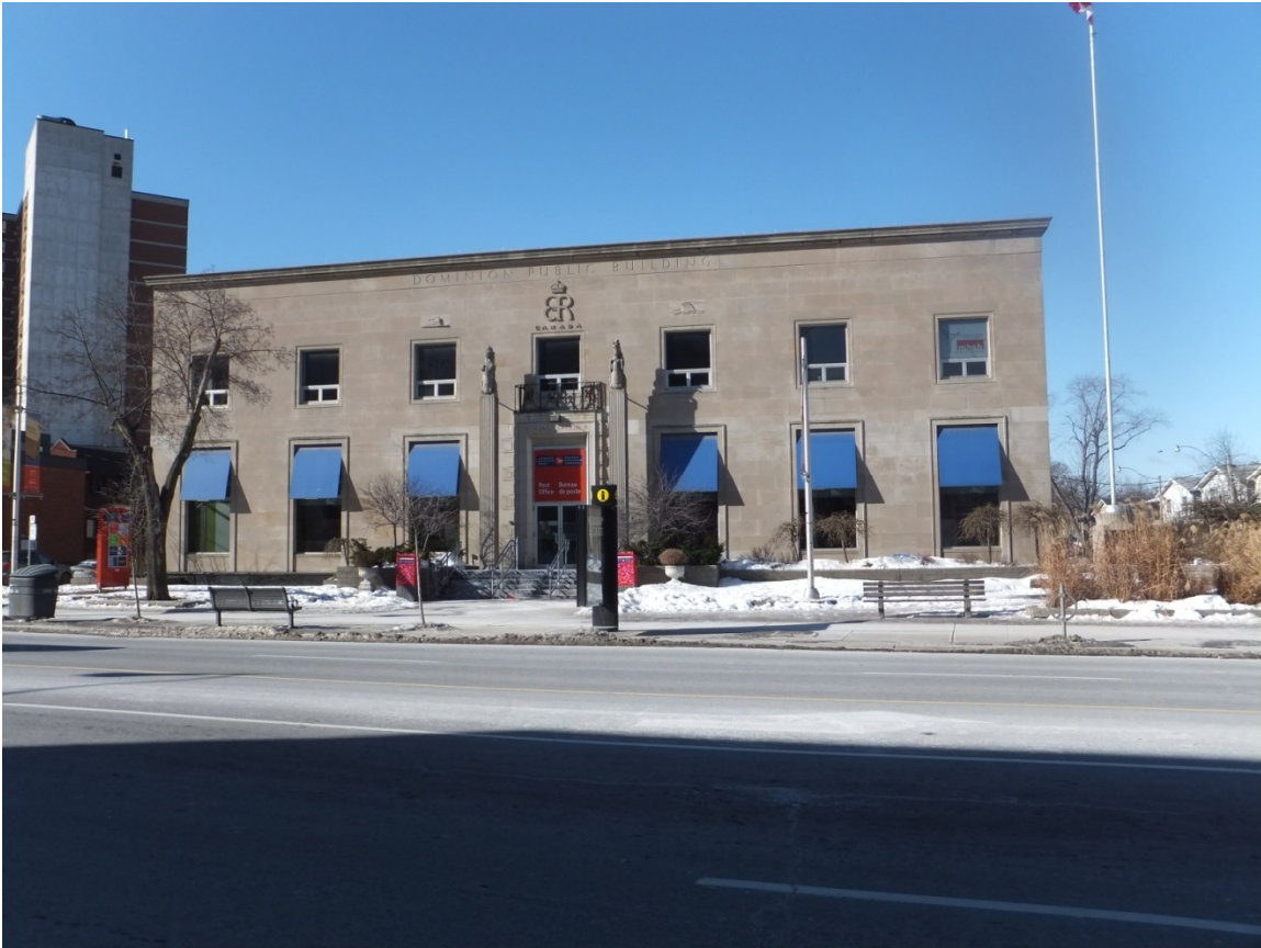
Photograph of the existing front elevation
