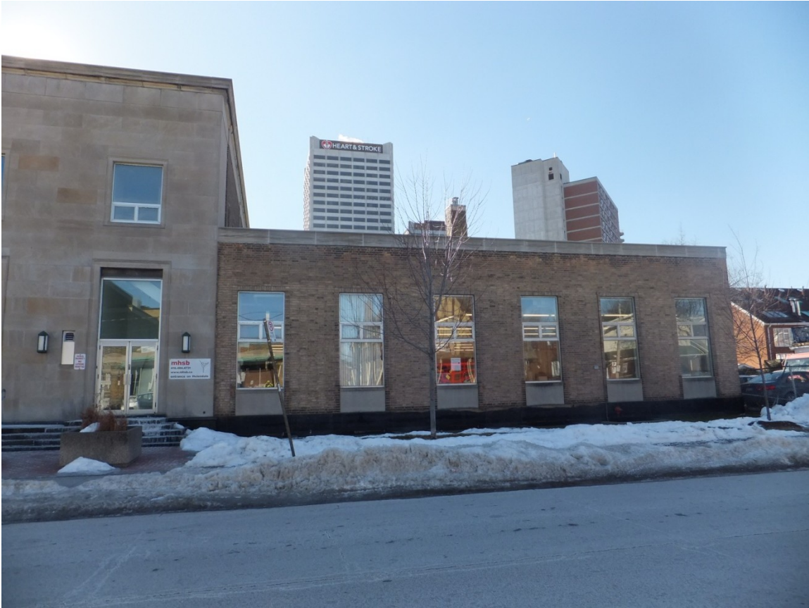
Photograph of the existing rear elevation
