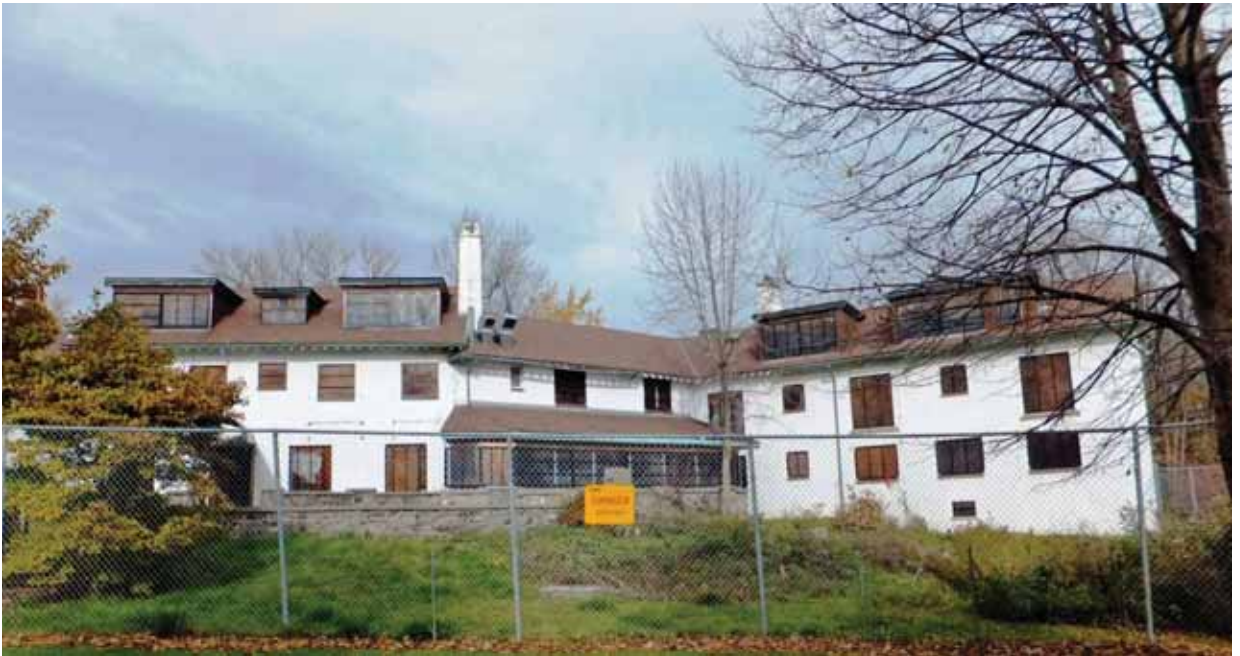
7.10. Bickford House, 2013: showing the north (above) and south (below) elevations
