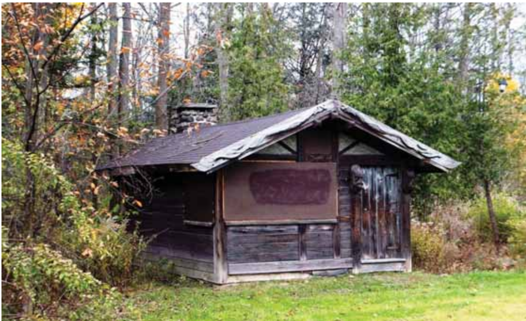
7.11. Sculpture Studio : showing archival and current images of the building with the sculpted detailing (the archival photograph is reproduced from Lidgold, The Guild Inn , 2000)
