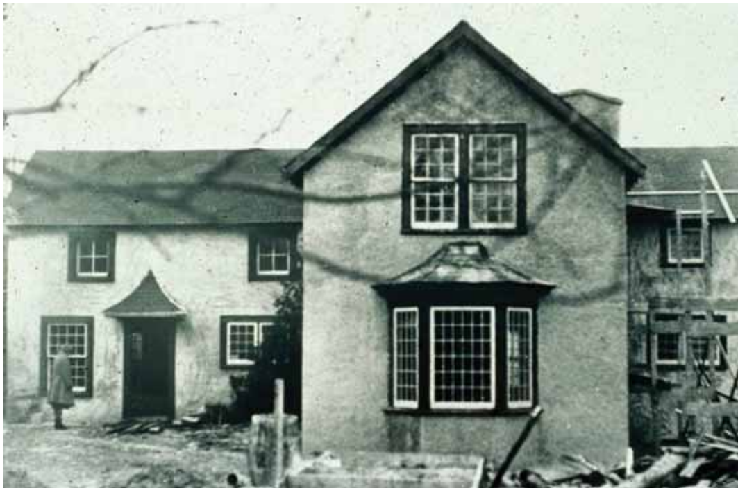
7.13. Studio Building : Constructed from outbuildings designed for the Ranelagh Park estate with a later addition, the structure was demolished in 2008 after extensive fire damage
