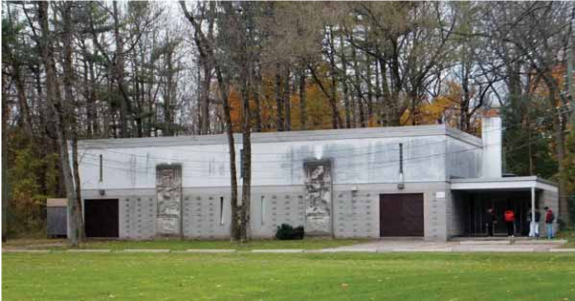
7.12. Building 191 : showing the building designed for Spencer Clark's art collection where the principal (east) facade incorporates the Marguetta Stone from the University Avenue Armouries and bas-reliefs from the Globe and Mail Building
