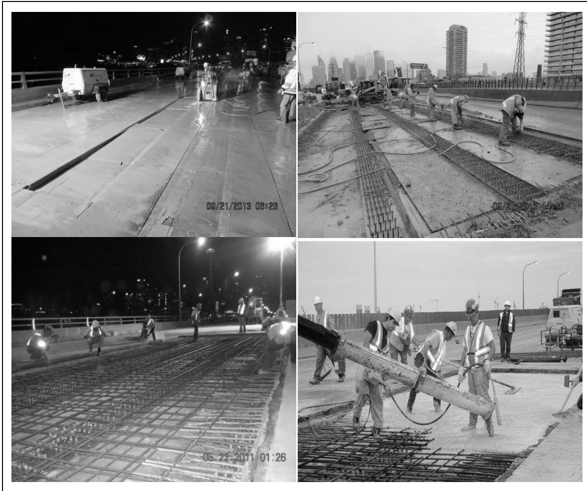
Figure 8: Photos of Deck Replacement Using Conventional Construction Methods
