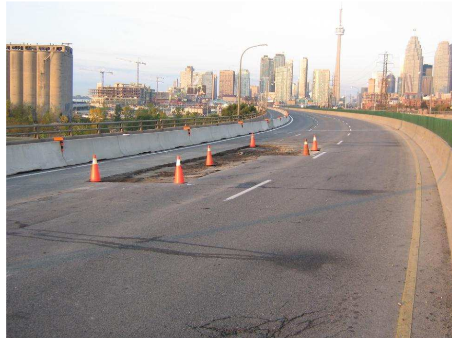
Photograph 1. - Showing removed Asphalt.
