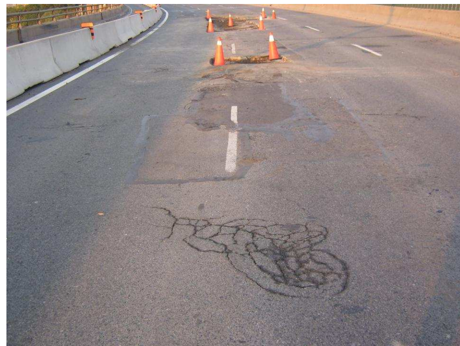
Photograph 2. - Showing removed Asphalt lanes 2 and 3.
