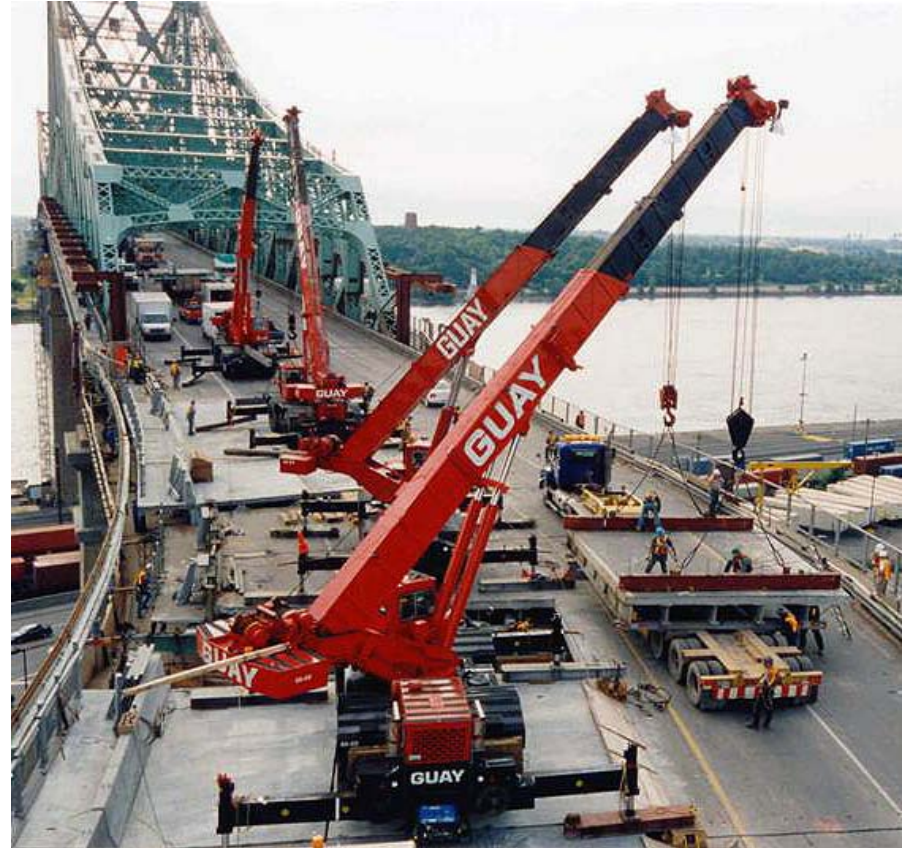
Placement of Prefabricated Deck-Girder Section
