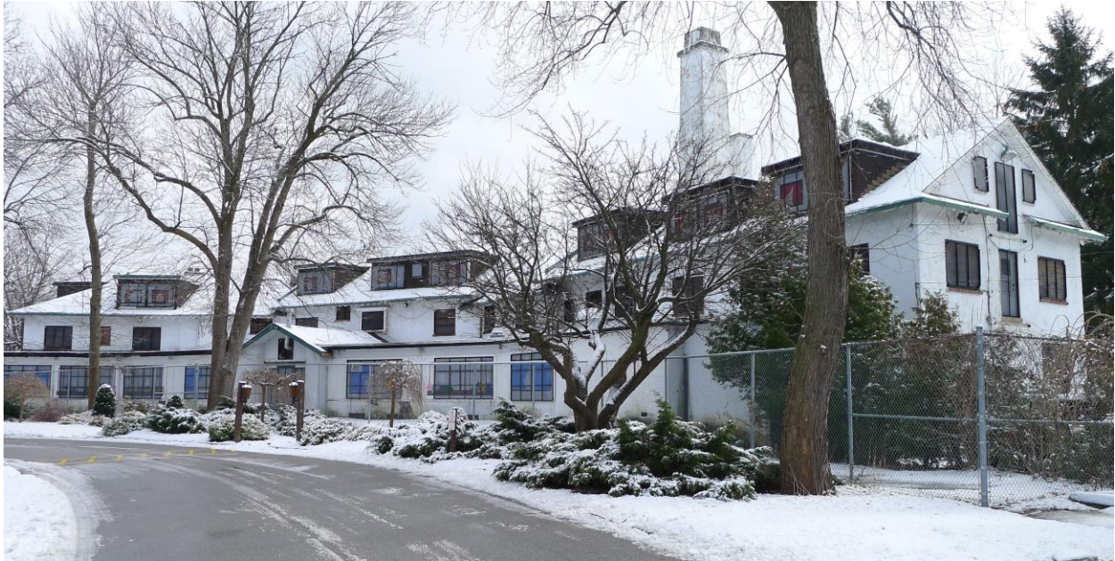
Bickford House, North Elevation, November 2013. The applicant is proposing to restore the Bickford House to its 1932 appearance. The lobby addition, later dormers, and east and west wings would be removed. The wood clad windows will be installed and the porte cochere will be restored.
