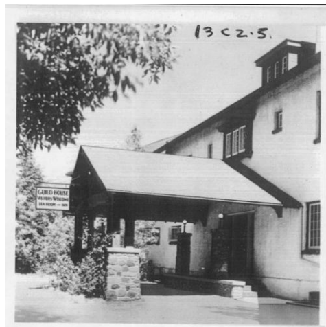
North Elevation of the Bickford House c. 1937 showing the original porte cochere.
