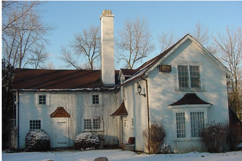
Studio Building December 16, 2002
