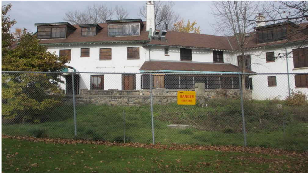
Bickford House, South Elevation, November 2013
