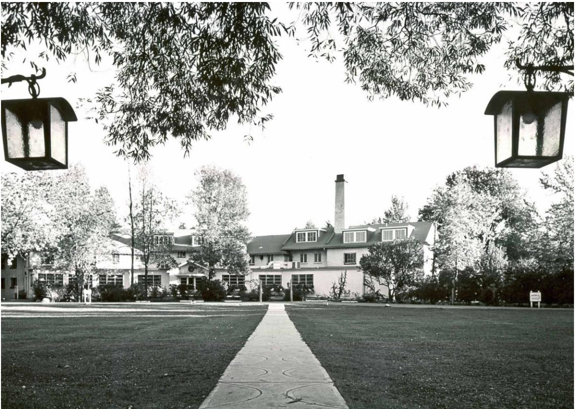
7.7. Archival Photographs, Bickford House : showing the north facade with the additions, including the dormer windows
