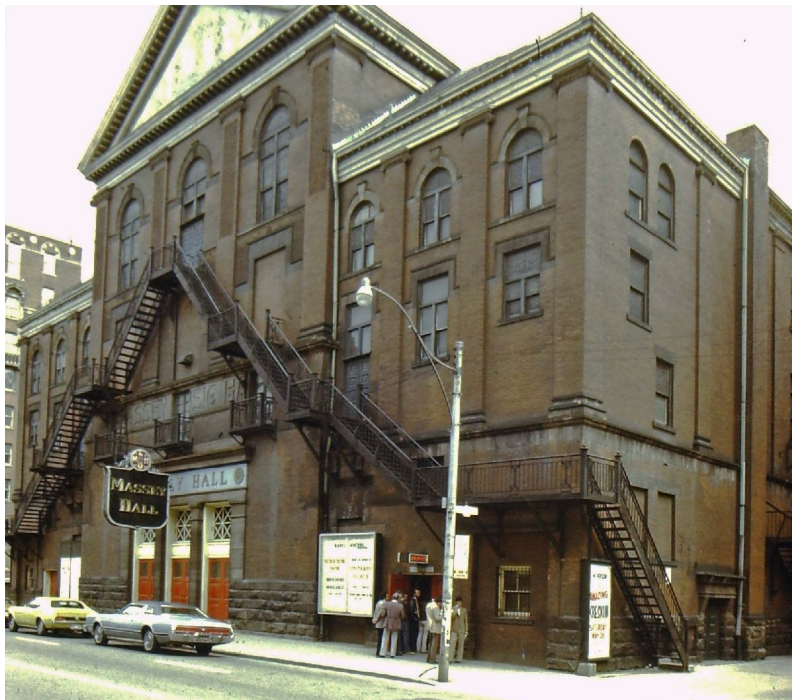
22. Archival Photograph, Massey Hall, c. 1973: showing the north facade at the time the property was listed on the City's heritage inventory (Toronto Historical Board)
