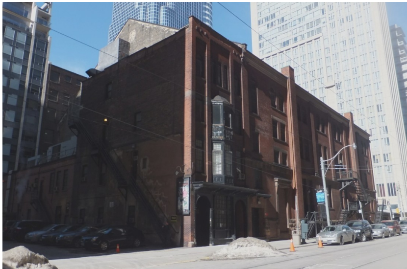
29. Current Photograph, Massey Hall : showing the east elevation on Victoria Street (right) and the rear (south) wall (left) with the two-storey Annex on the extreme left. The four-storey Albert Building is attached to the south wall (centre) (Heritage Preservation Services, 2013)
