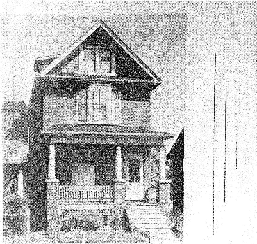
37 BOULTON AVENUE The House with the Red Doors
