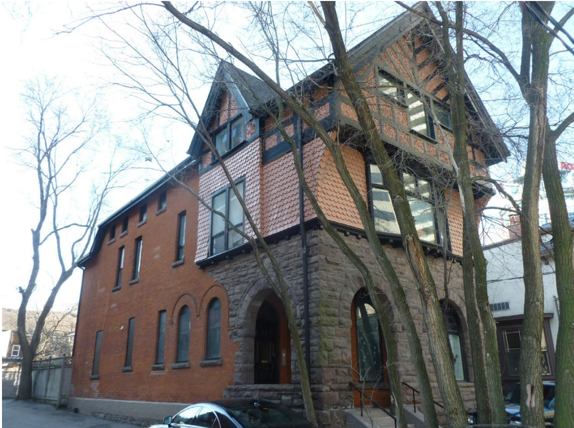
15 Selby Street, (A.H. Rundle House) north and east elevations
