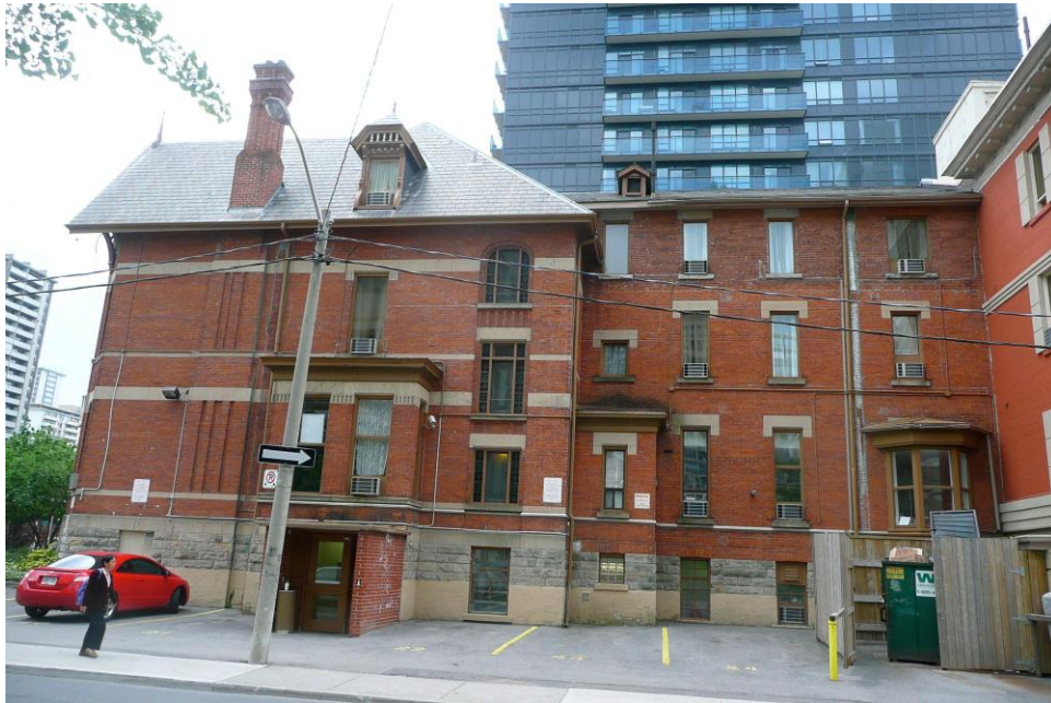
592 Sherbourne Street, North Elevation showing the house and the original inset 2 ½-storey rear-wing that would be altered
