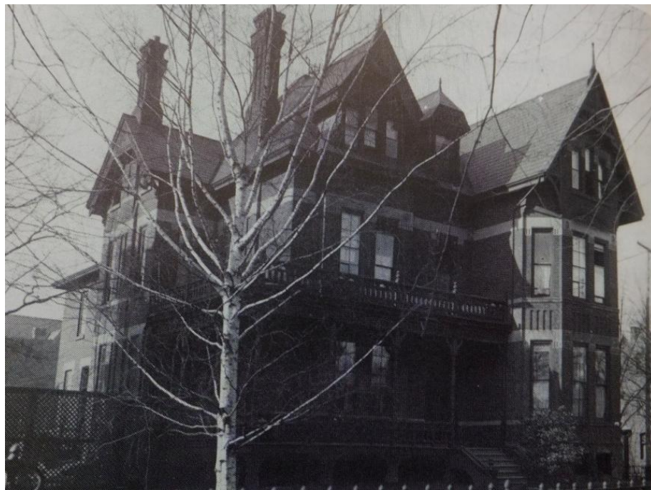
14. Archival Photograph, 1903 : showing the property prior to the death of C. H. Gooderham (Robertson, 22)
