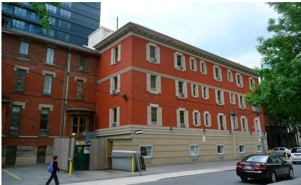
592 Sherbourne Street, North Elevation showing the four storey 1913 hotel addition that would be demolished
