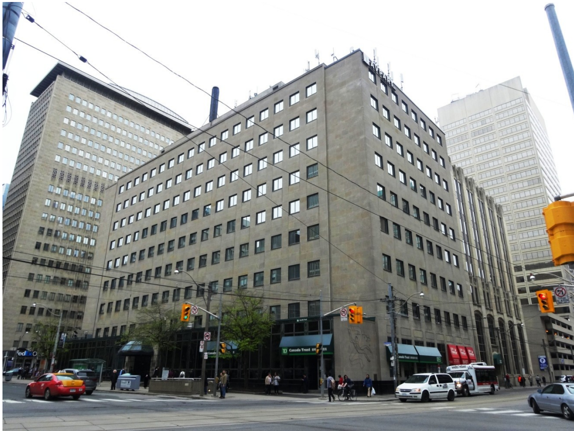
481 University Avenue (South and West Elevations)
