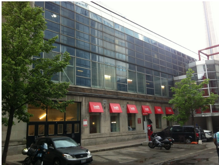
Remaining Stone Clad of Ground Floor of 7 Station Street
