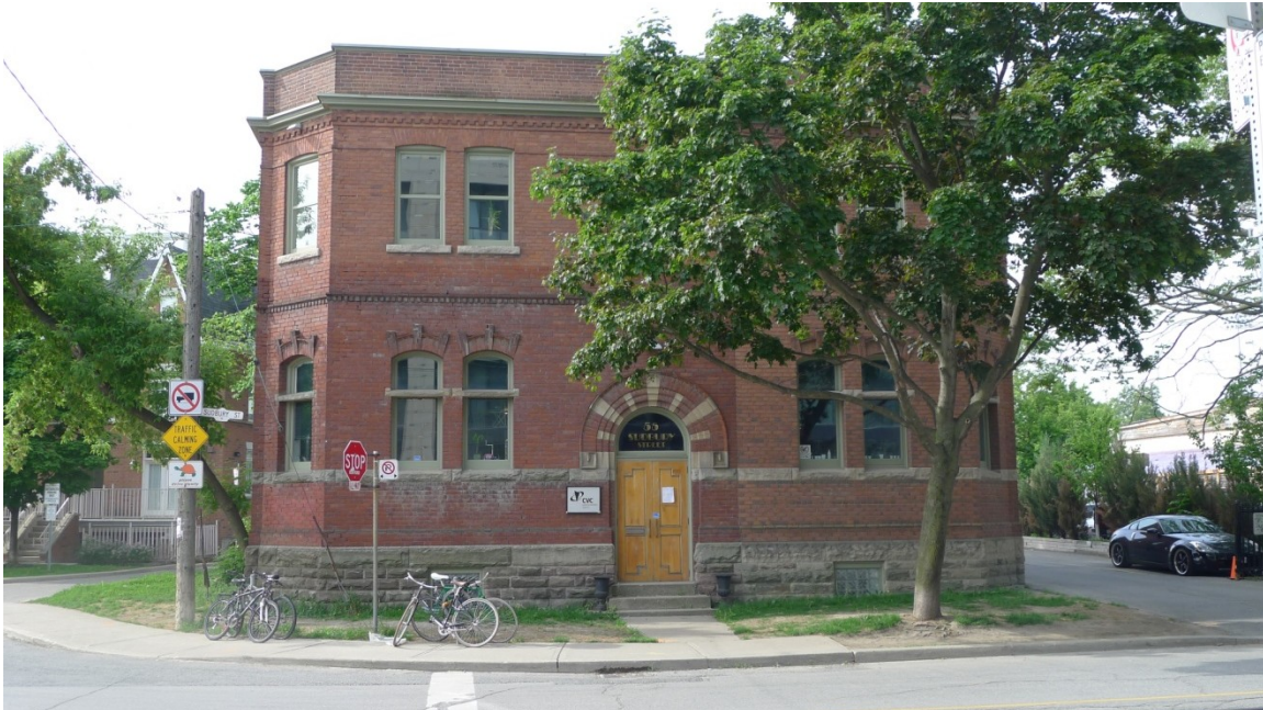
Above: principal (north) façade of the former Diamond Glass Company office building (Heritage Preservation Services 2014)
