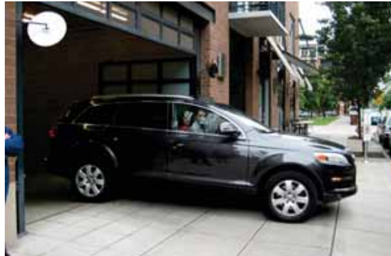
Figure 6.10 - Parking entries integrated into architecture
