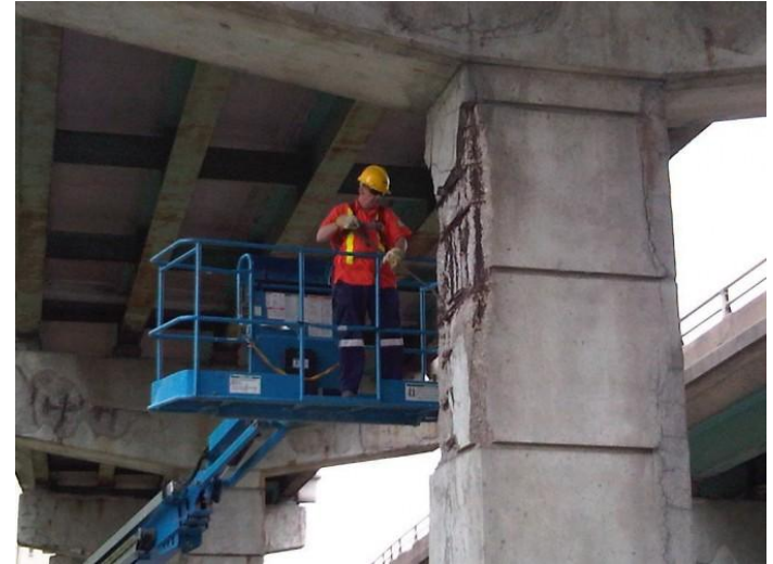
Controlled chipping work
