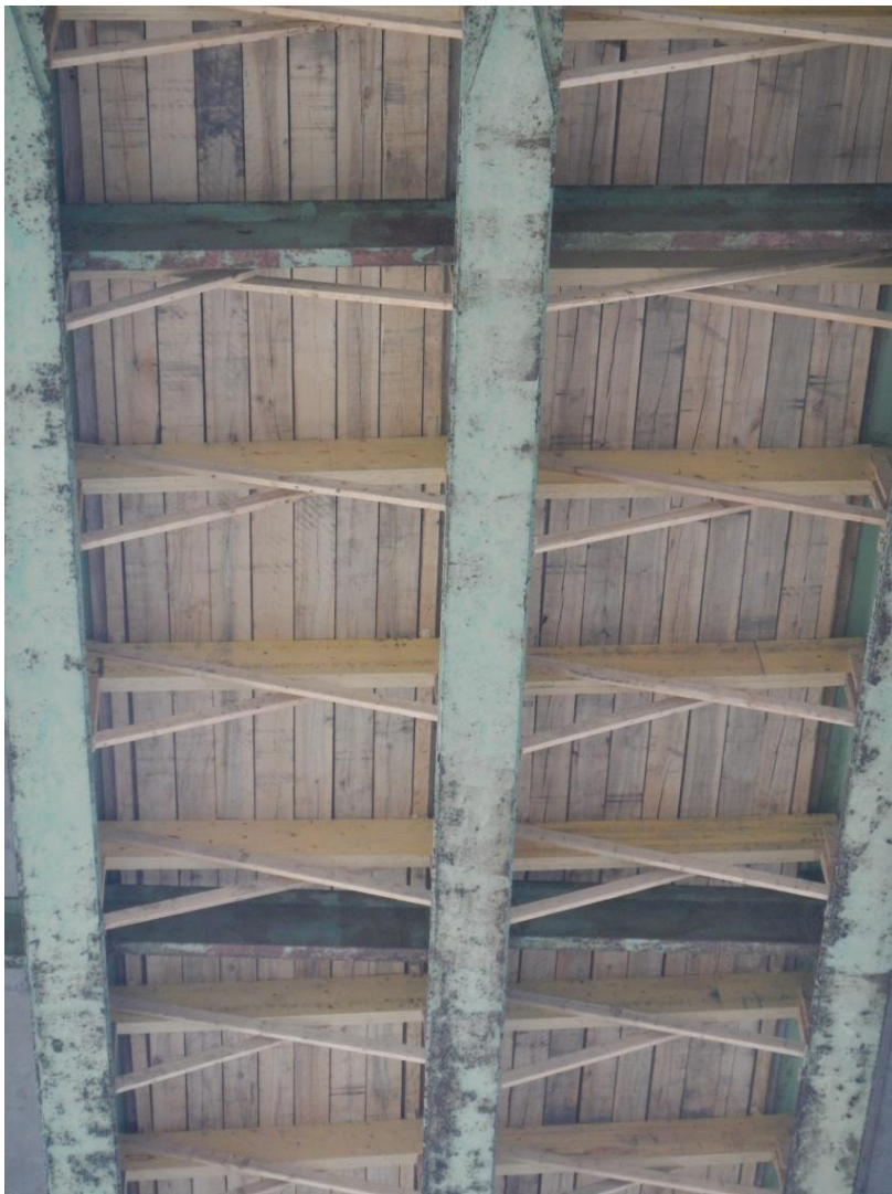
Deck shoring with timber bracing
