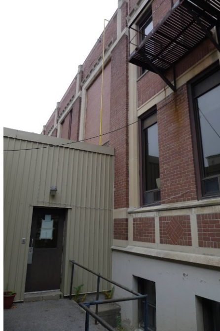
150 Laird Drive, west elevation, looking south, with the one-storey metal clad addition and the link to the main building (left) and, looking north, showing the link and the bricking in of the window at the second floor above the link (right) (HPS, 2015)
