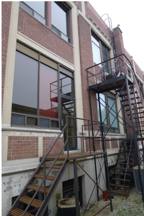
150 Laird Drive, west elevation, north end, showing the alteration to the window to accommodate exit door, addition of chimney and fire escape stairs (left) and with another view of the fire escape stairs, various railings to basement access and other alterations (right) (HPS, 2015)
