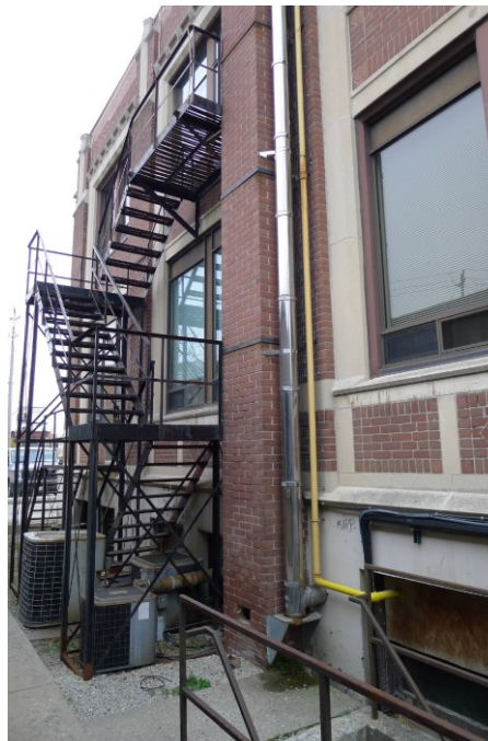
150 Laird Drive, west elevation, north end, showing the alteration to the window to accommodate exit door, addition of chimney and fire escape stairs (left) and with another view of the fire escape stairs, various railings to basement access and other alterations (right) (HPS, 2015)
