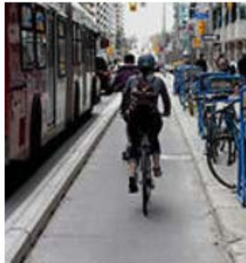
Cycle Track separated by curb stones.
