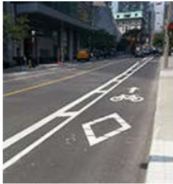
Buffered bike lane— paint only.
